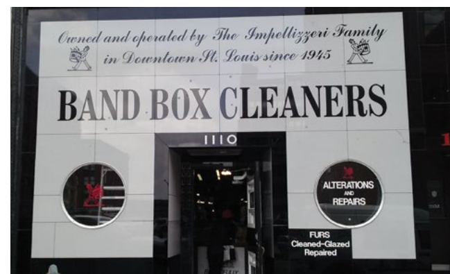
[14] The signage is an original and integral part of this historic Carrara glass storefront.
