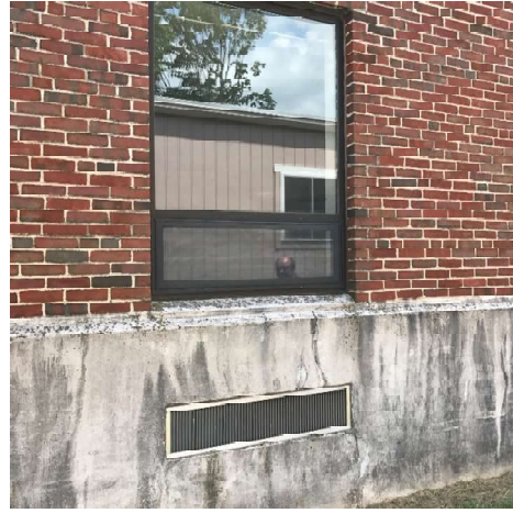
Figure 17—Non thermally broken windows
