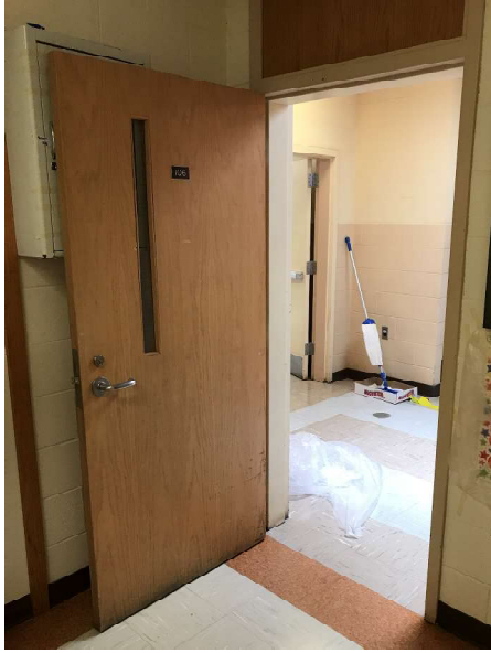
Figure 60—Typical natural finish wood door
