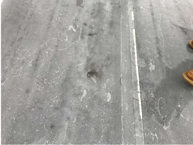
Figure 31– Visible scrim layer on '52 building roof
