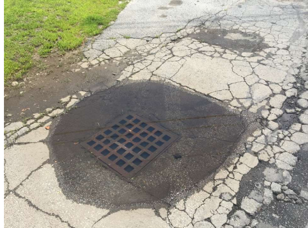
Figure 28—Catch basin at drop-off loop
