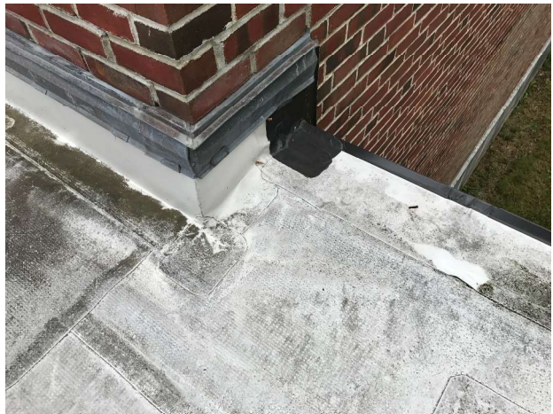
Figure 34– Undulating flashing on '83 addition roof
