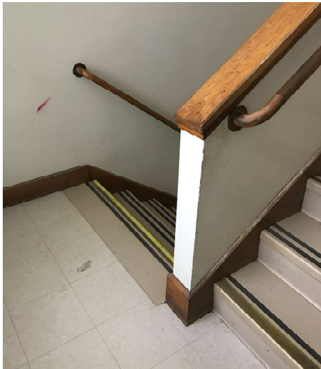
Figure 18—Typical egress stairwell handrails
