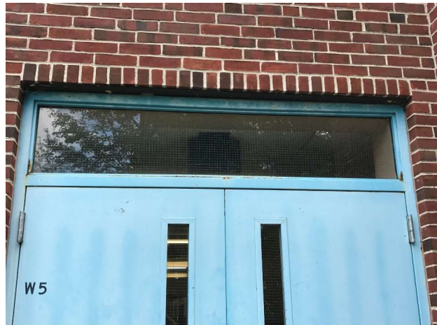
Figure 25—Exterior hollow metal doors
