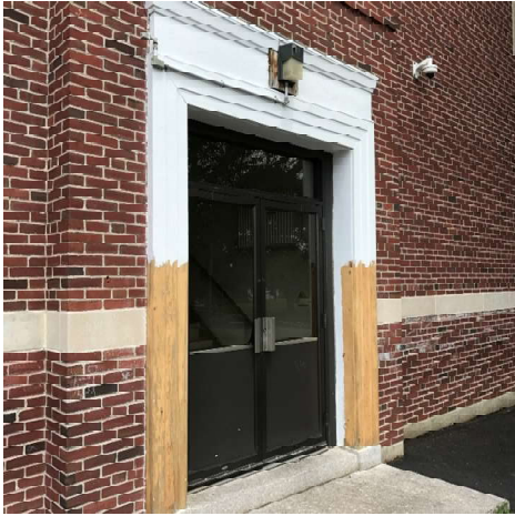
Figure 22—Storefront door at '52 building
