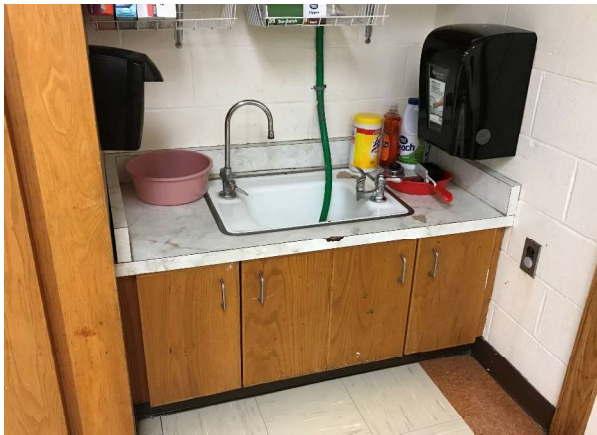
Figure 66—Classroom casework sink base
