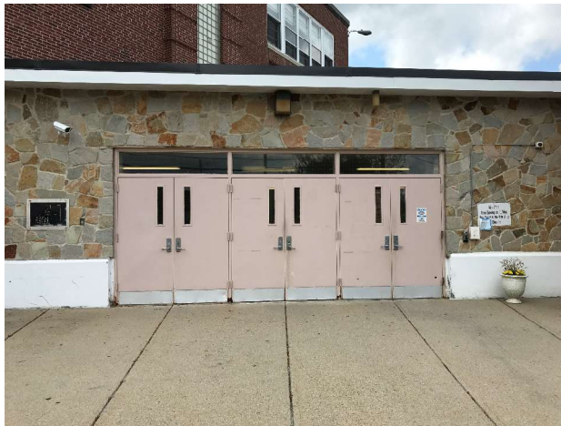
Figure 3—Main entry doors
