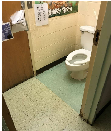
Figure 13—Non-accessible toilet in nurses suite
