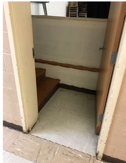
Figure 8—Stair at side of stage / platform
