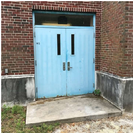
Figure 24—Exterior hollow metal doors
