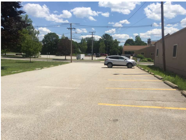
Figure 29—Parking at school.
