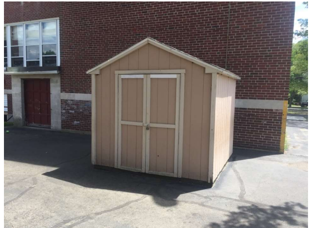
Figure 12—Storage shed at playground
