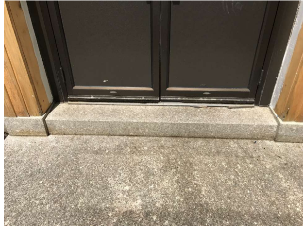
Figure 23—Storefront door at '52 building
