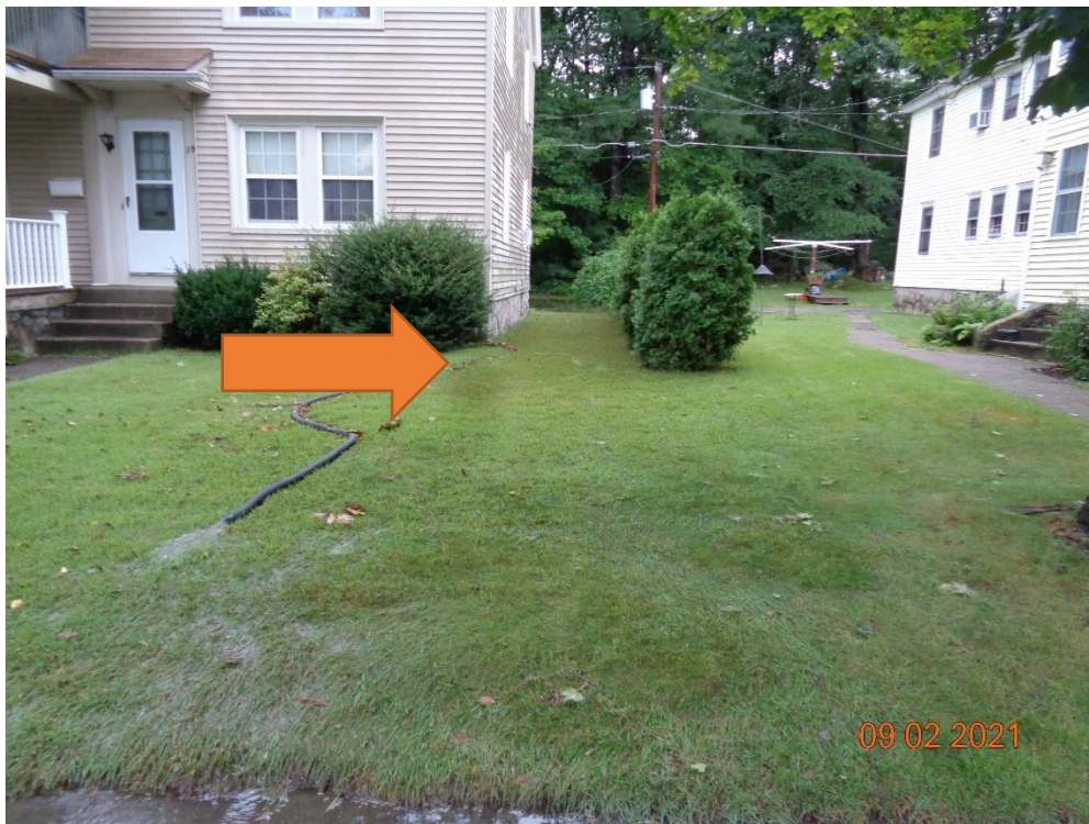
Photo 2: Flooding in the backyard of #19 Leland Road. The arrow points to evidence (leaf litter) that the water level rose to the point that water flowed overland from the backyard.
