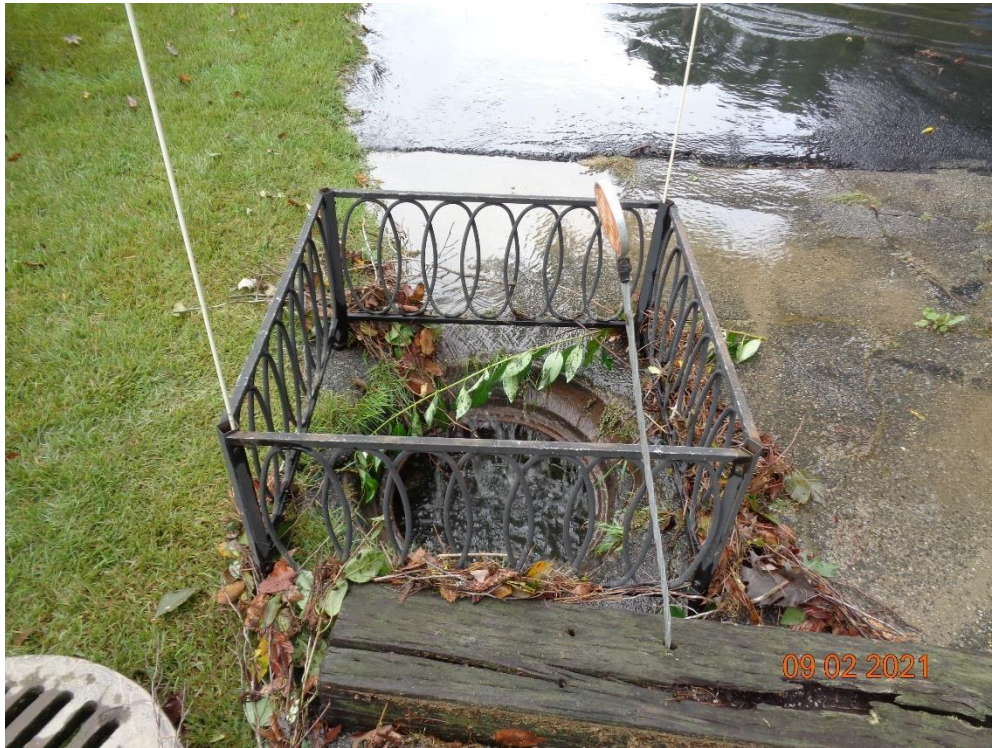
Photo 5: Catch basin between #19 and #21 Leland Road.
