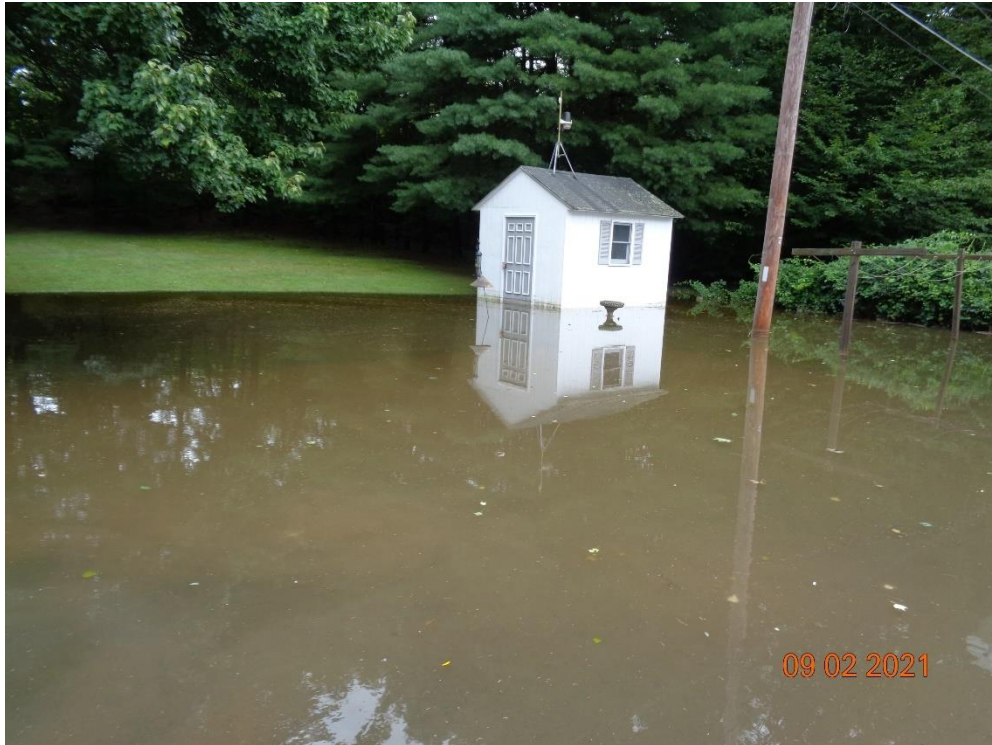
Photo 1: Flooding in the backyards of #15 and #17 Leland Road.
