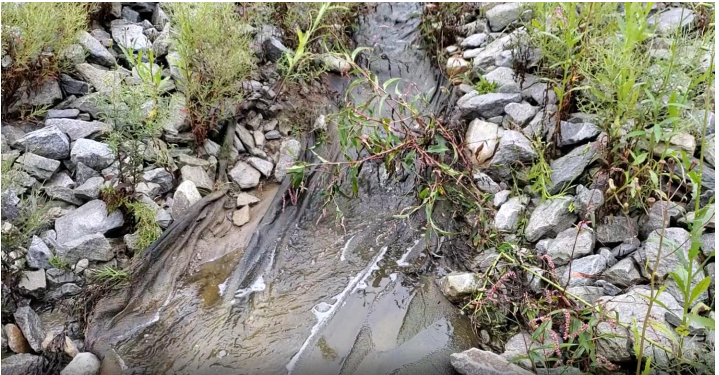
Flow from the access road drainage swale entering into Area 9
