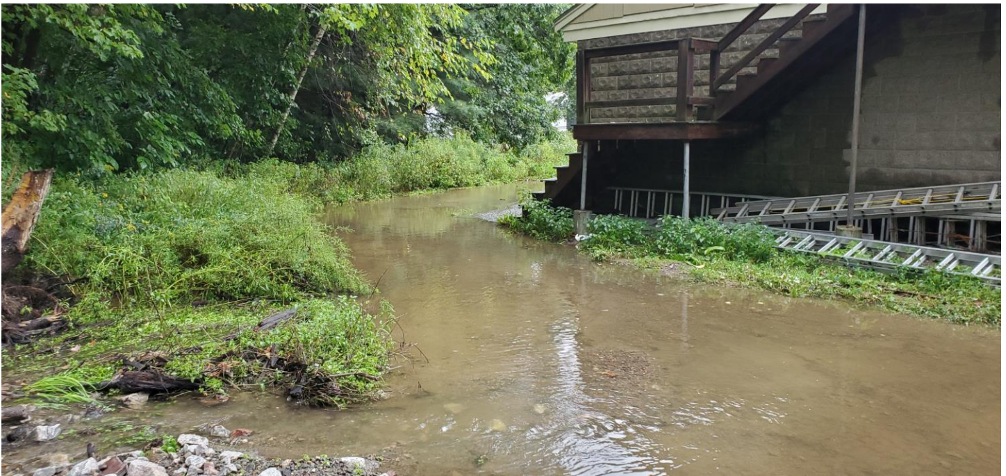
View of water flowing through breach in berm around garage towards Area 1
