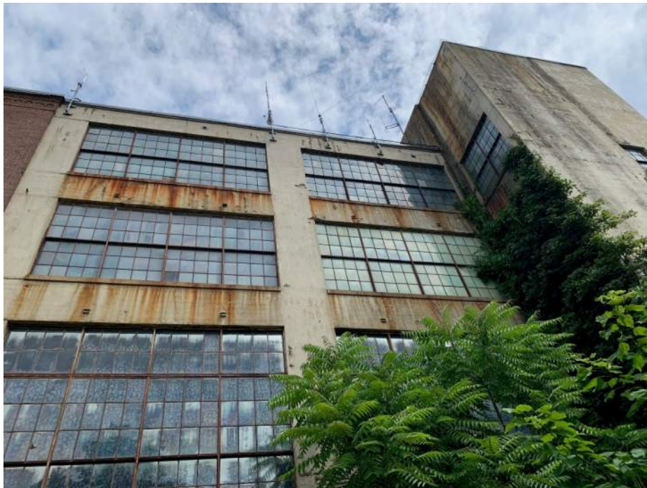
Photo #12: Overall view of rear elevation of building.
