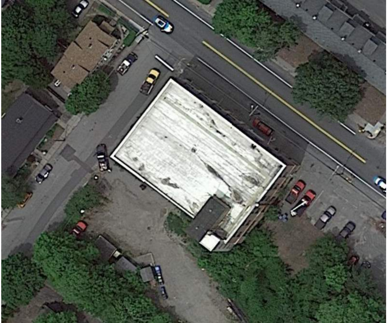
Photo #1: Aerial view of subject building (via Google Earth).
