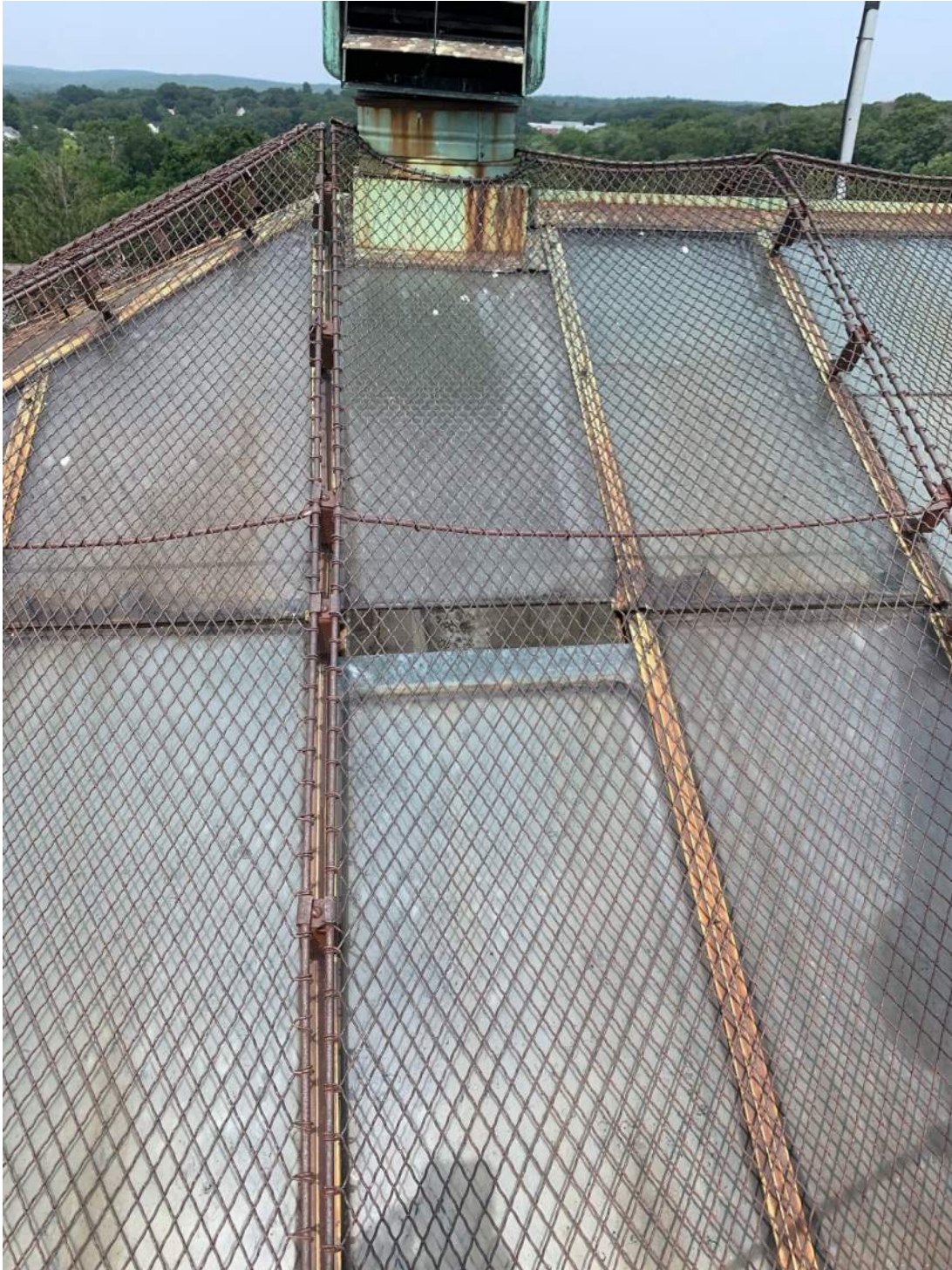
Photo #9: Close-up view of opening in glazing system above freight elevator.
