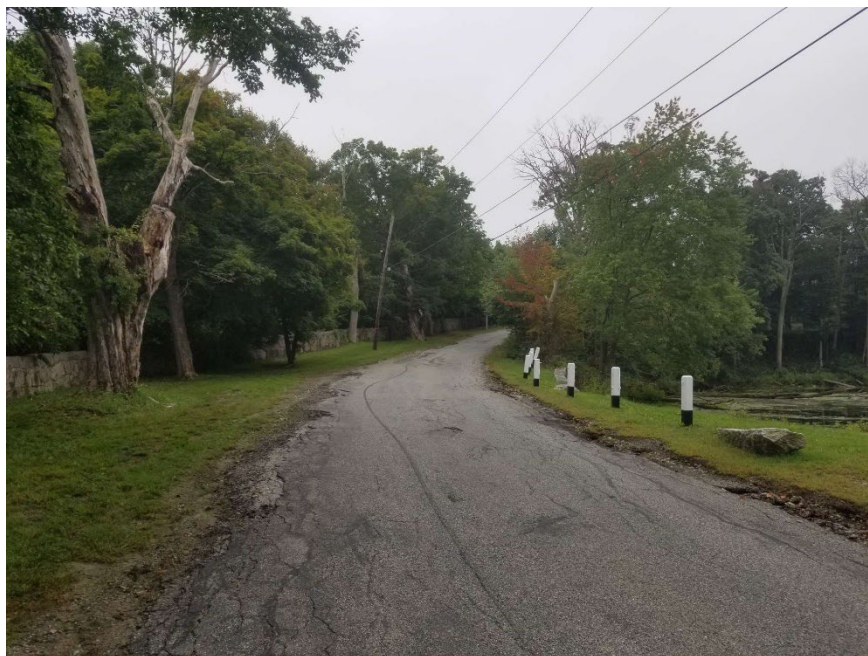
Street Scene Looking Southerly Along Castle Hill Road.
