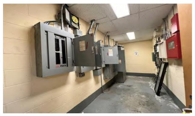
Photo 29: Electrical room in the central portion of Building 1 (facing south). Electrical panels appeared to be in good condition.
