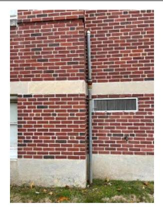
Photo 20: Approximately 2-inch vent pipe associated with the abandoned UST (facing west).
