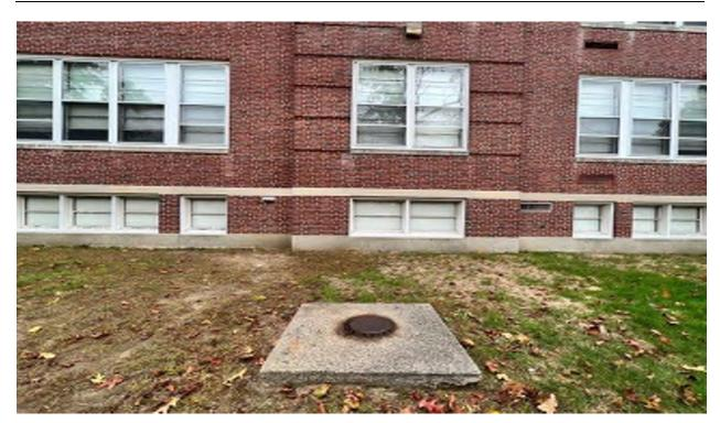
Photo 18: Abandoned underground storage tank (UST) located to the east of Building 1 (facing west).
