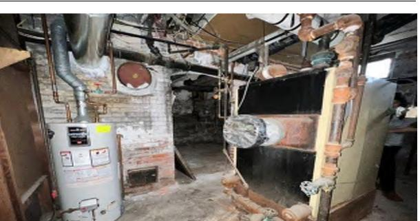
Photo 42: Former boiler and new hot-water boiler located in basement of Building 2 (facing north). Note de minimis staining surrounding boilers on concrete flooring.
