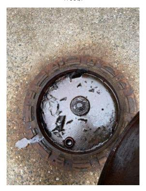
Photo 19: Fill port and rainwater observed beneath the manhole cover of the abandoned UST (facing west).
