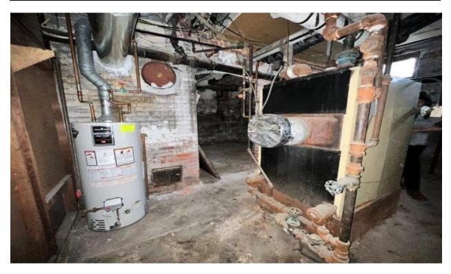
Photo 42: Former boiler and new hot-water boiler located in basement of Building 2 (facing north). Note de minimis staining surrounding boilers on concrete flooring.
