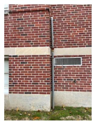
Photo 20: Approximately 2-inch vent pipe associated with the abandoned UST (facing west).
