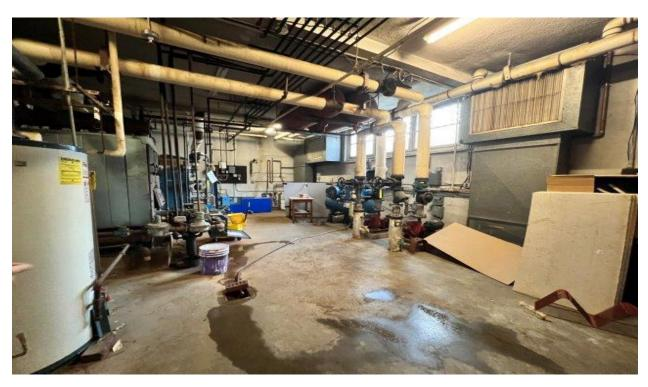
Photo 34: Mechanical/boiler room located in the southwestern portion of Building 1 (facing northwest). Floor drains are connected to the municipal sewer system.
