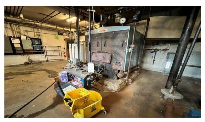
Photo 36: Former boiler located in mechanical/boiler room in the southwestern portion of Building 1 (facing south).
