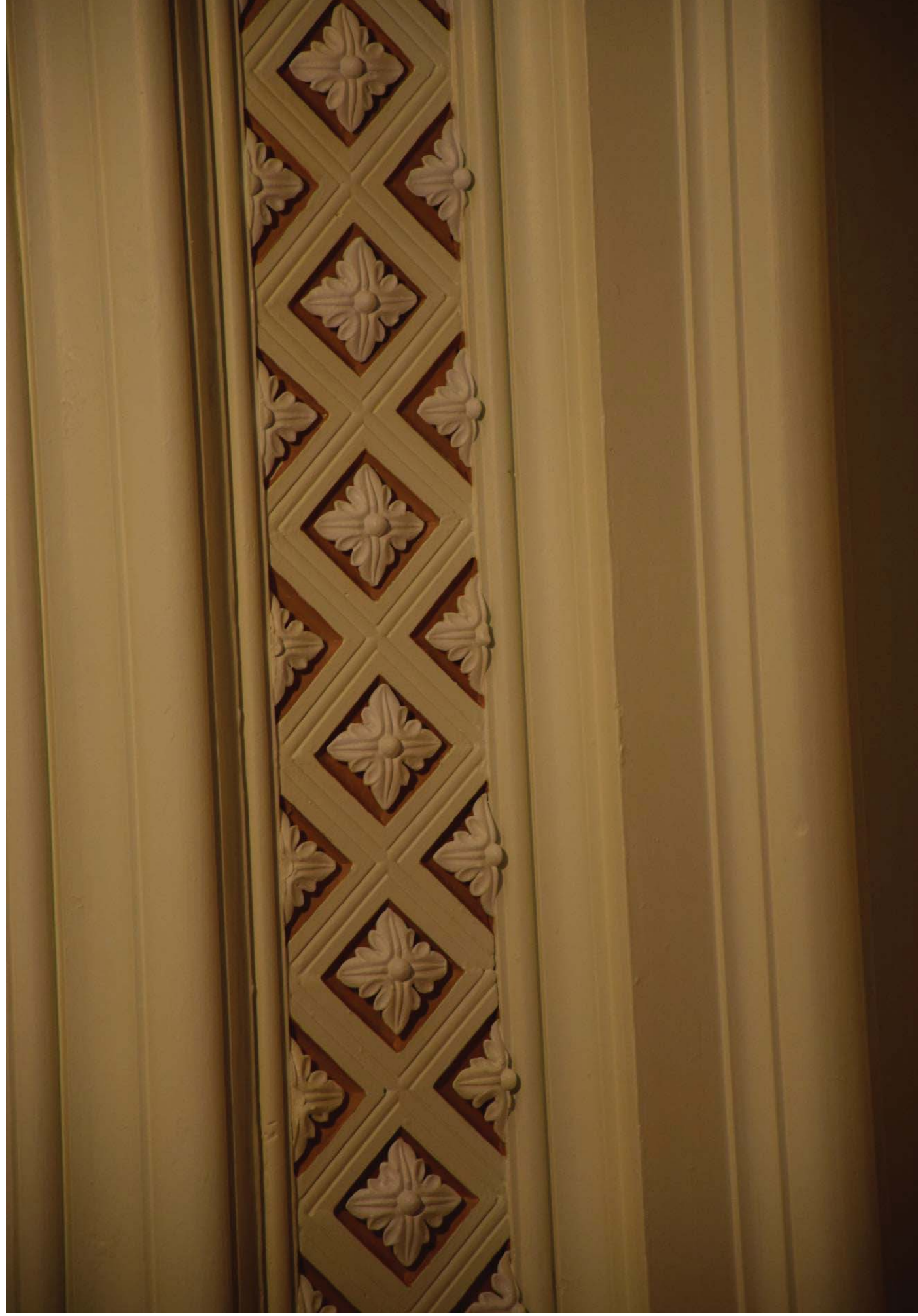
17. Close-up view of small ceiling cove bosses.
