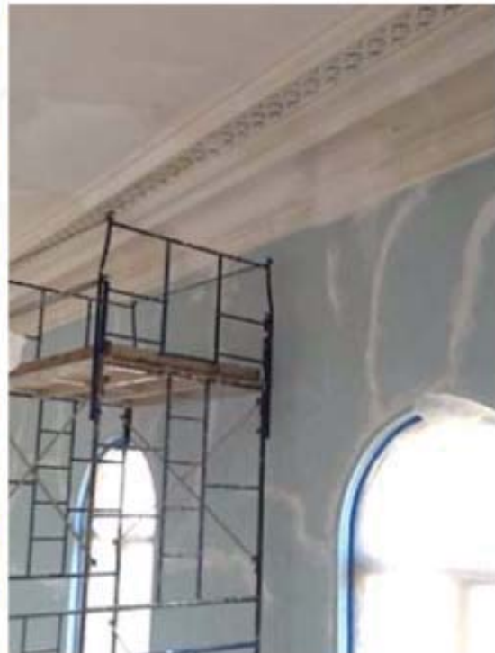
Crown molding and cracked plaster need a lot of attention.
