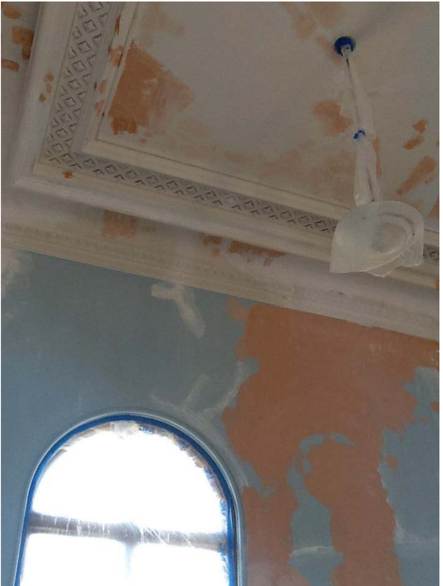
8. Paint preparation work in progress.
