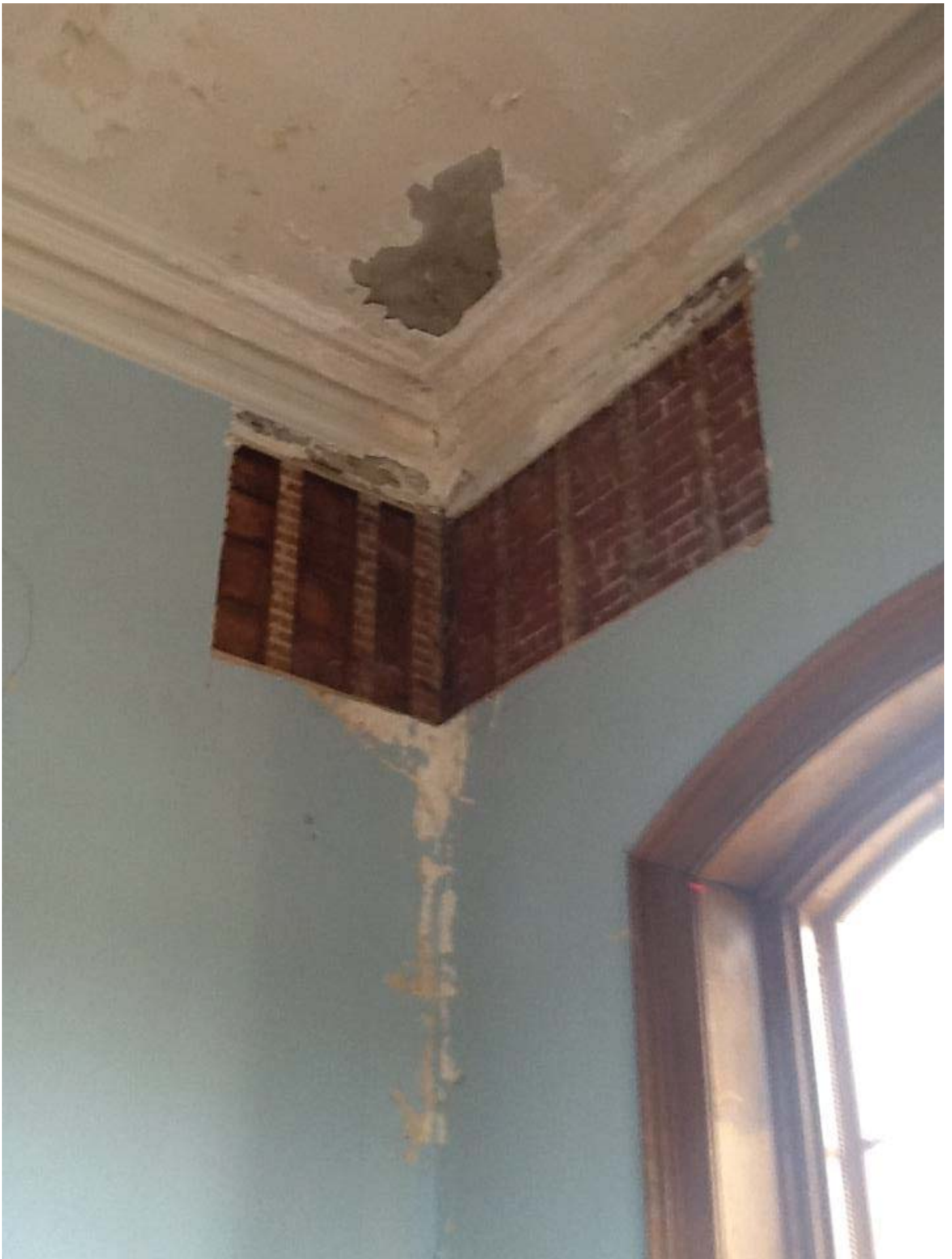
5. This section of asbestos containing plaster was removed by the abatement contractor. Full containment was first constructed to contain all AMC containing dust.
