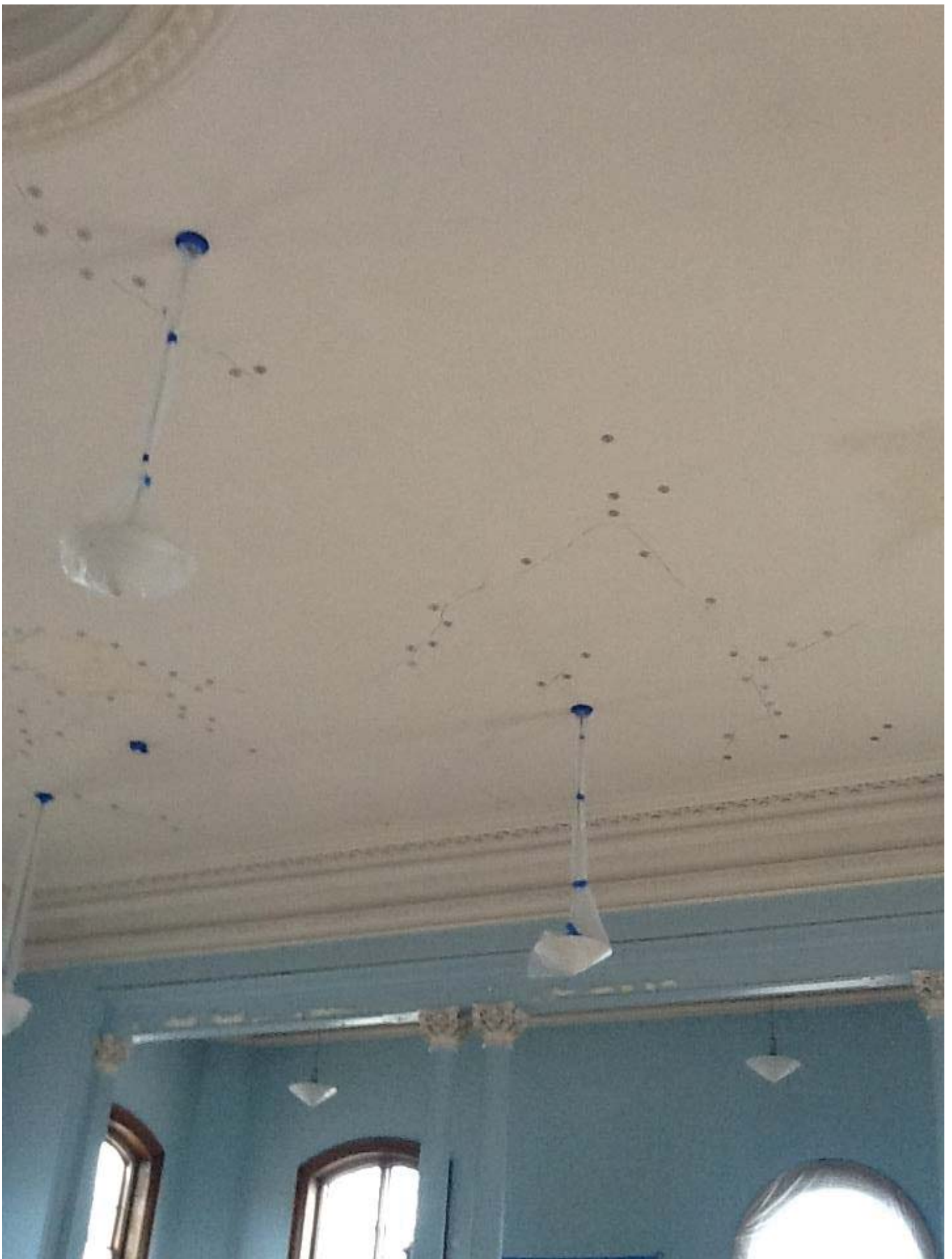
4. Temporary “button” can be seen, which are used to hold the plaster in place while the adhesive that secures the loose plaster to the wood lath dries.
