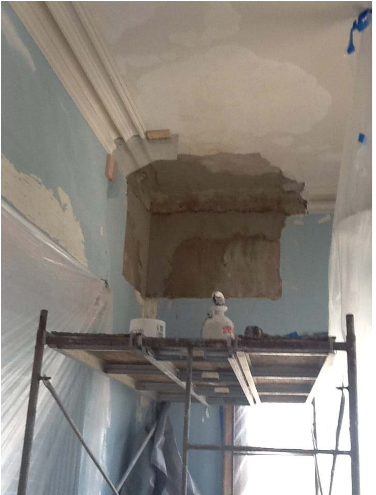
6. Scratch coat of plaster applied to wall area which have been abated and area of deteriorated ceiling plaster.
