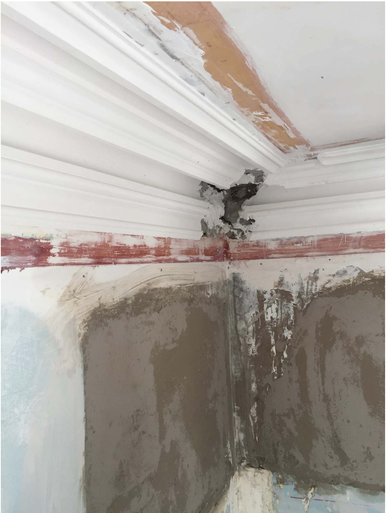
7. This section of asbestos containing plaster was removed by the abatement contractor. Full containment was first constructed to contain all AMC containing dust.
