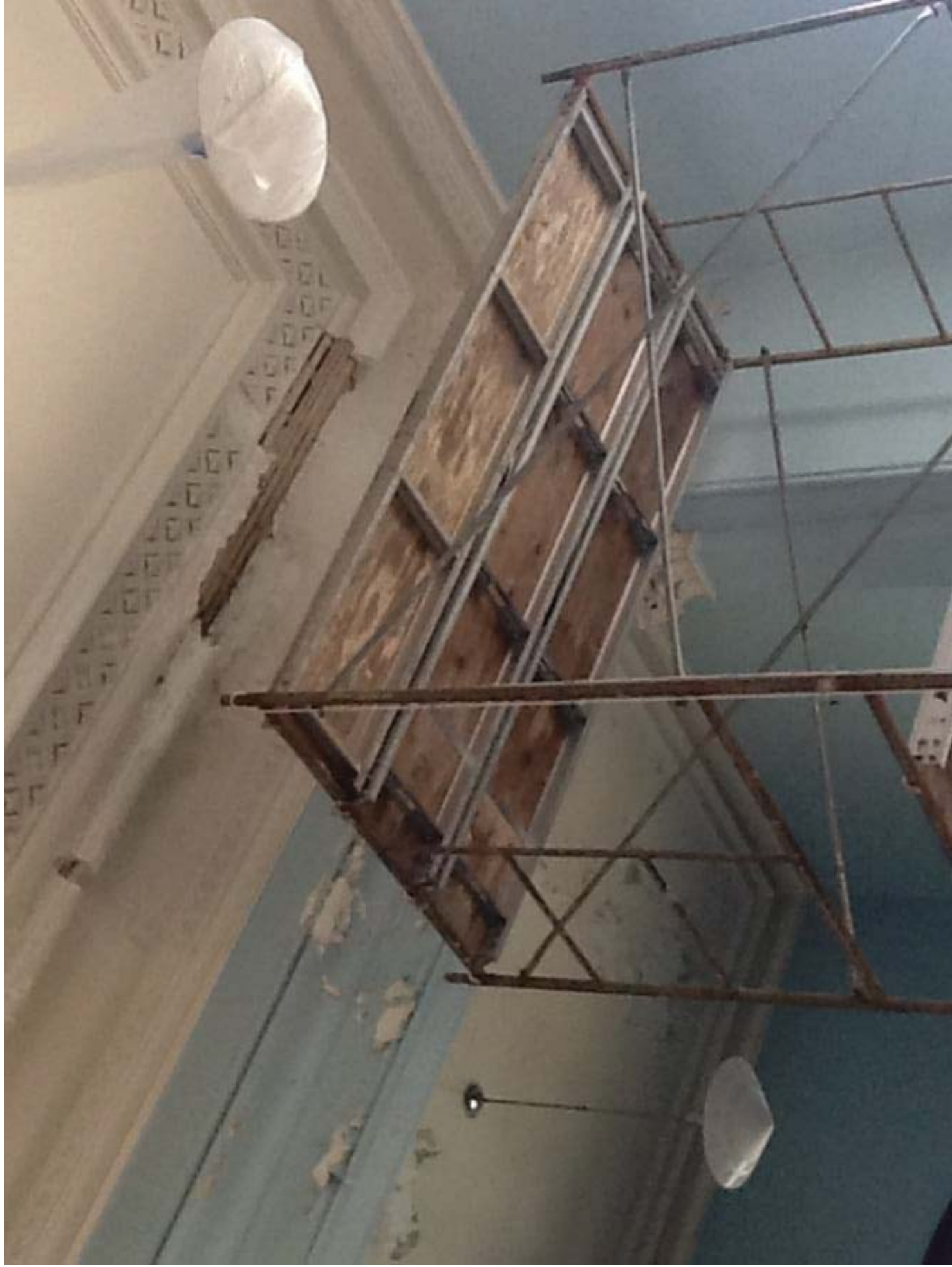
1. View of Great Hall ceiling cove, showing deterioration.
