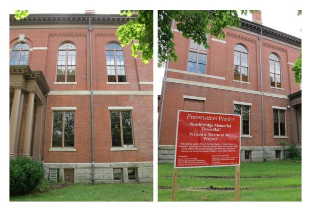
On the exterior, painting of the window frames is underway, weather permitting. The window sills on the south side of the building (parking lot side) have required a fair amount of epoxy consolidation and patching of the weathered sill surfaces. The north side (Main Street side) window sills were in much better shape, and required much less work. The new storm windows, as well as the new windows at the south side of the basement, should be arriving during the week of July 22nd.
