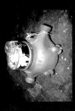
Whitinsville Water Company Existing meters are positive displacement piston style meters As water passes through meter, piston moves causing meter head to spin
