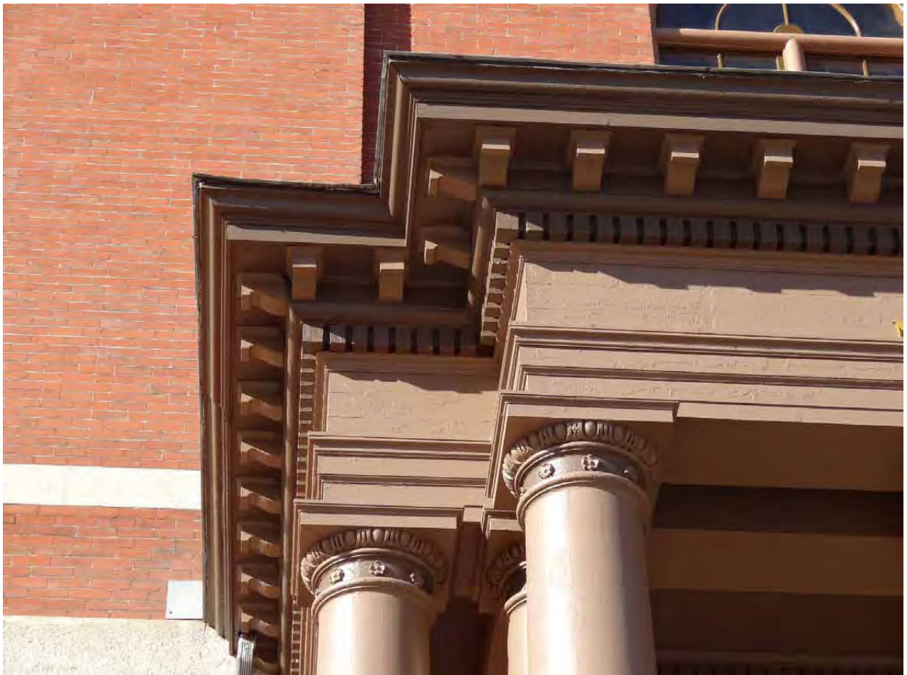
11. Restored East Portico Cornice and Columns
