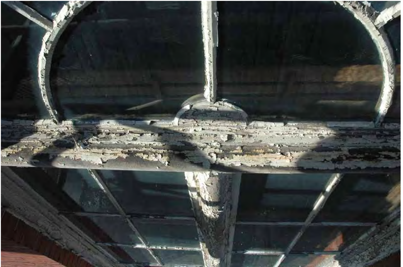
12. 2012 photograph of typical window with failed glazing putty and sealants at window perimeters and failed paint.
