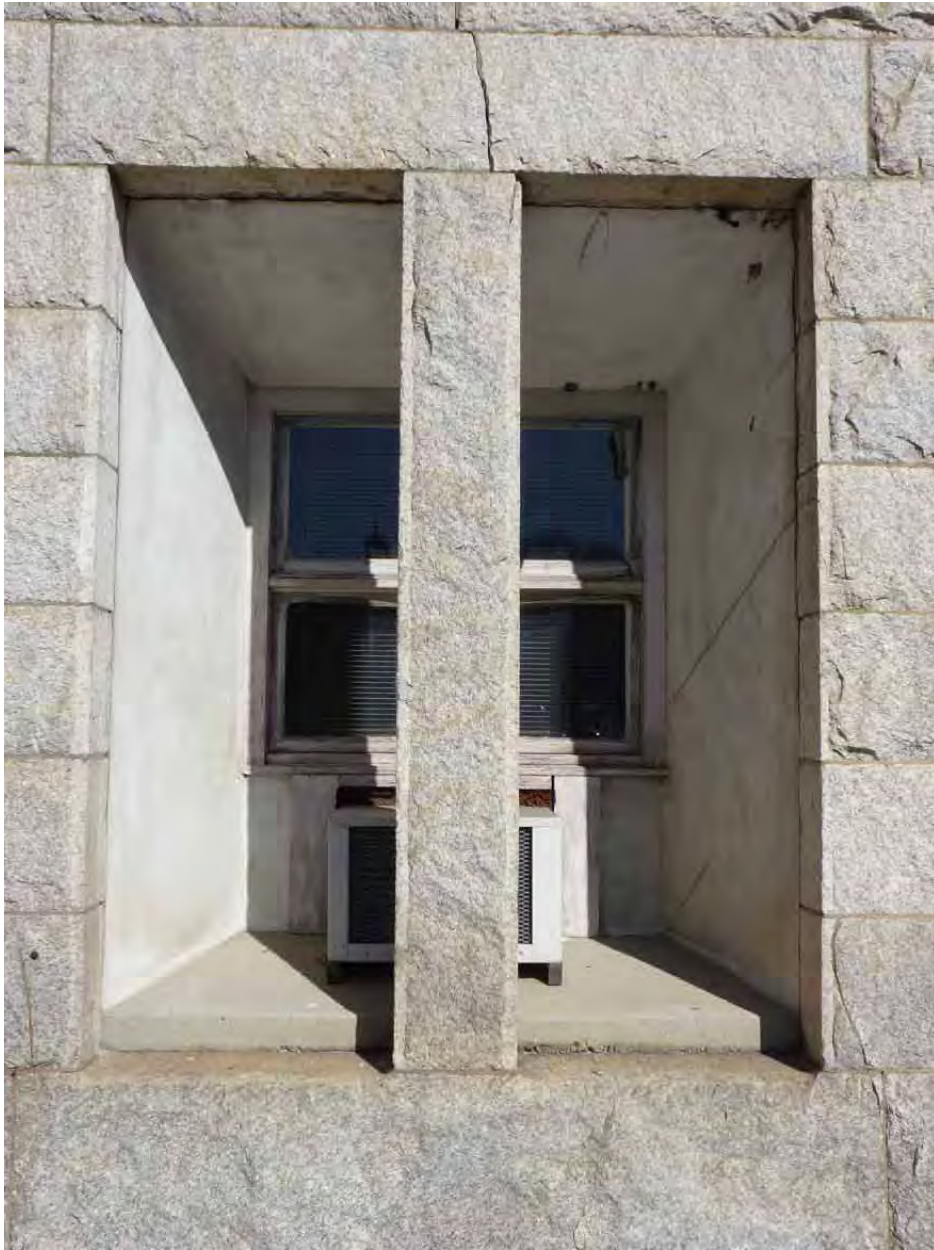
33. Ground Floor Replacement Window and Air Conditioning
