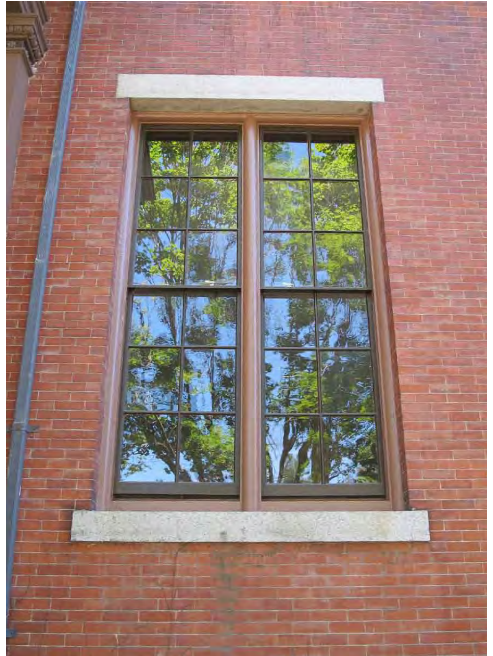
32. Restored window: The operation of the restored window sashes is relatively easy, considering that the sash weights only exist at the masonry opening side of each window, and not within the central vertical mullion. The narrow proportions of the new windows probably make this possible.
