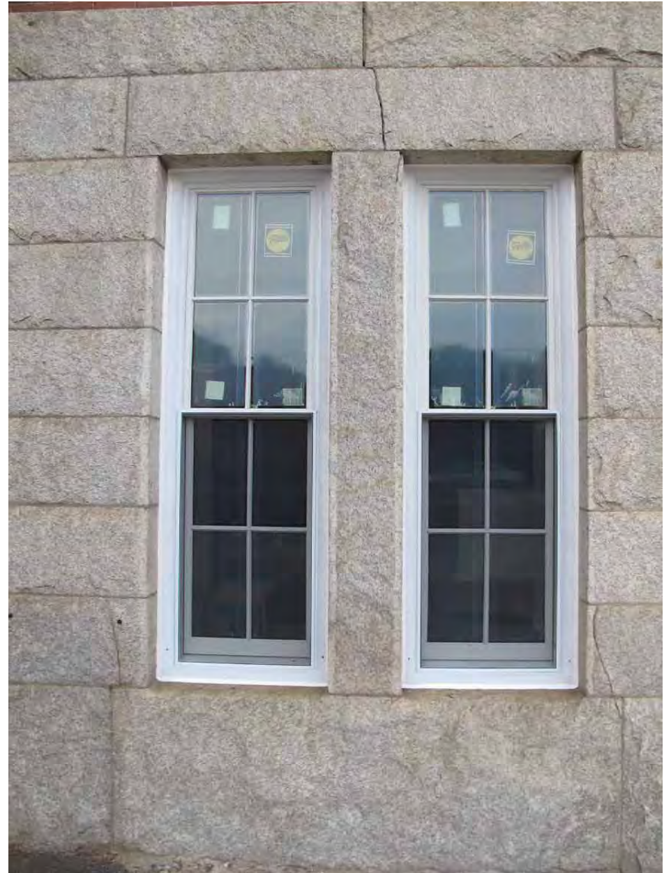
34. Construction Photo Showing Replica Historic Windows Prior to Field Painting
