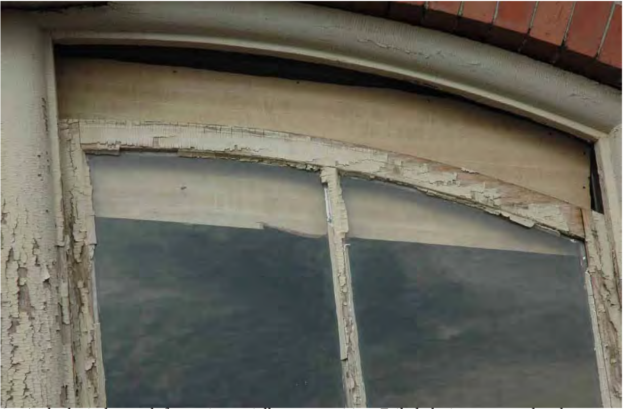
25. Arched window sash frozen in partially open position. Failed glazing putty and sealants at window perimeters also contributed to water and air infiltration.
