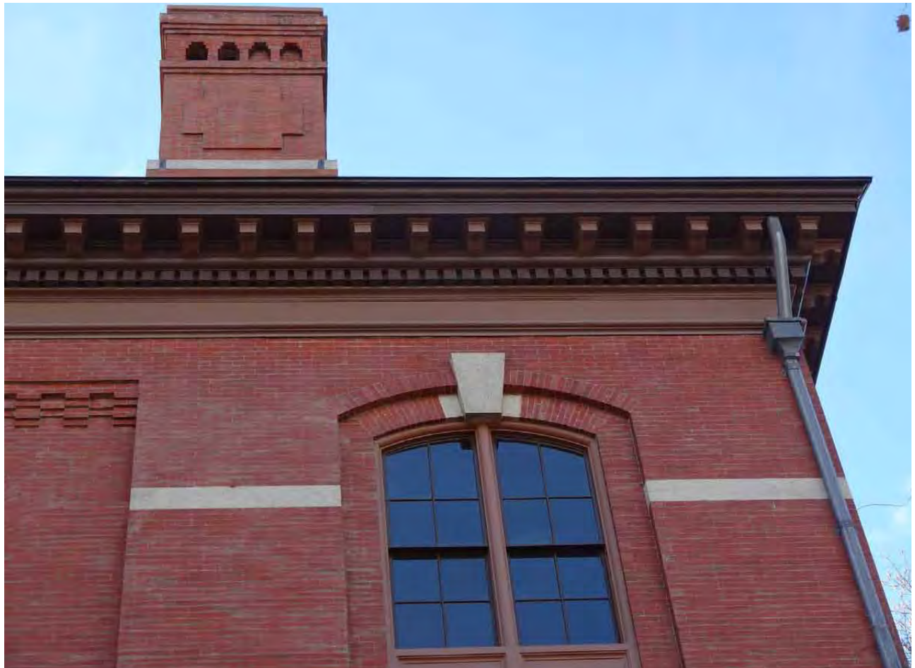
7. Restored Horizontal Cornice and Windows
