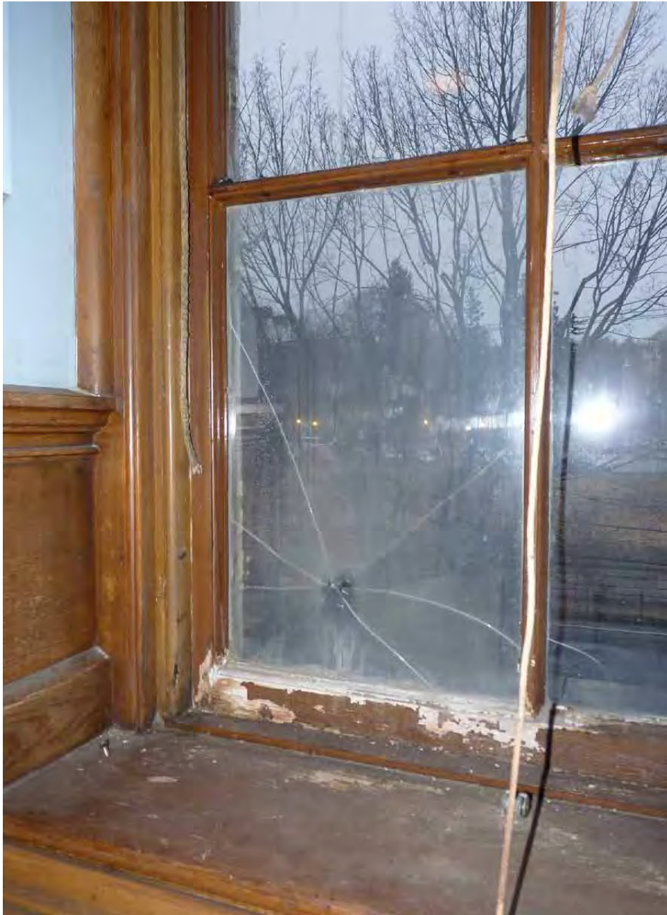
23. Typical First Floor Window (Interior): Window finish is water damaged due to missing glazing putty, sash cords are broken, and there is glass breakage.
