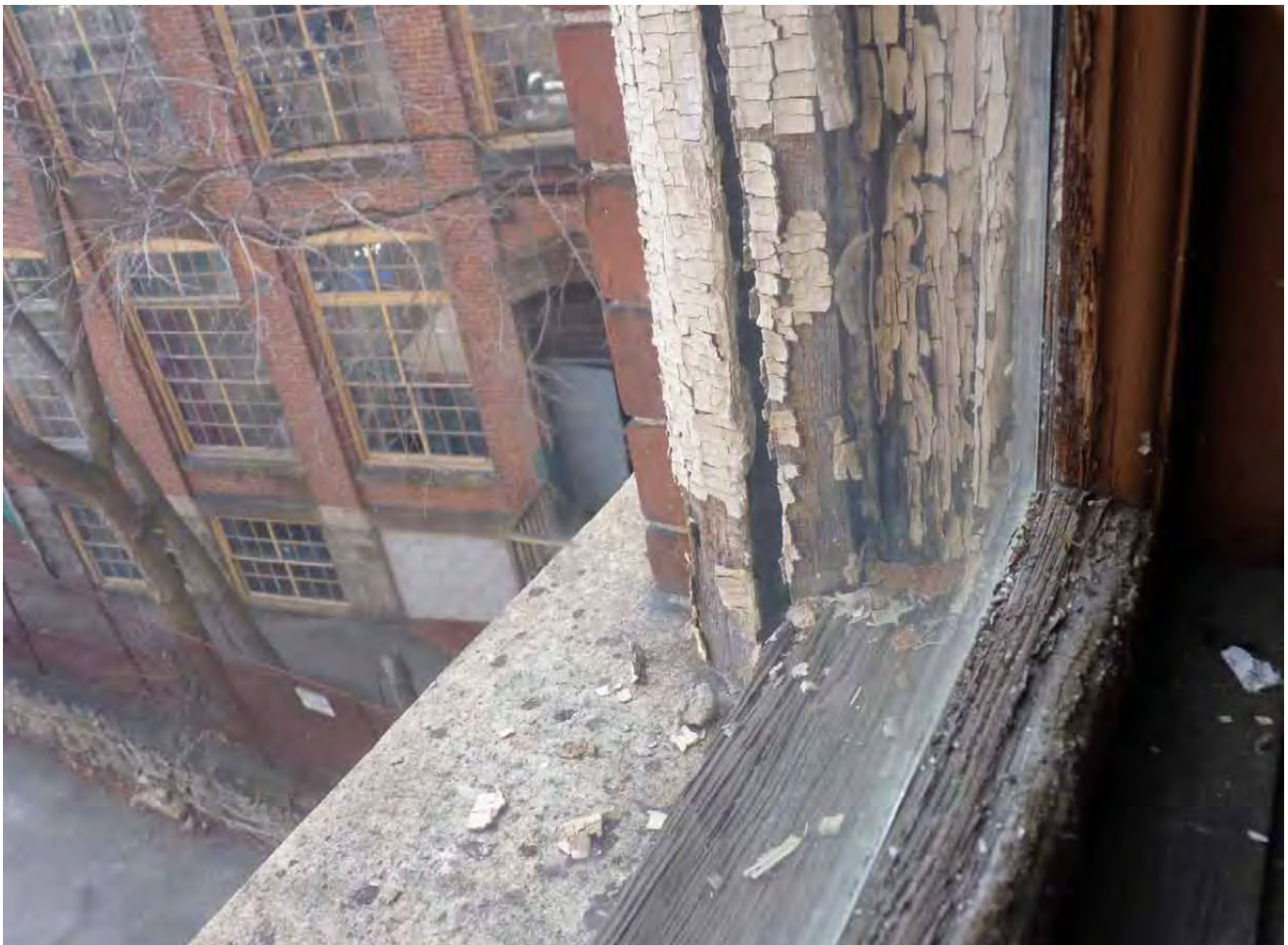
15. Sills on the south side of the building were much more deteriorated than the sills on the north side. Damaged sill surfaces were consolidated and patched with epoxy materials.
