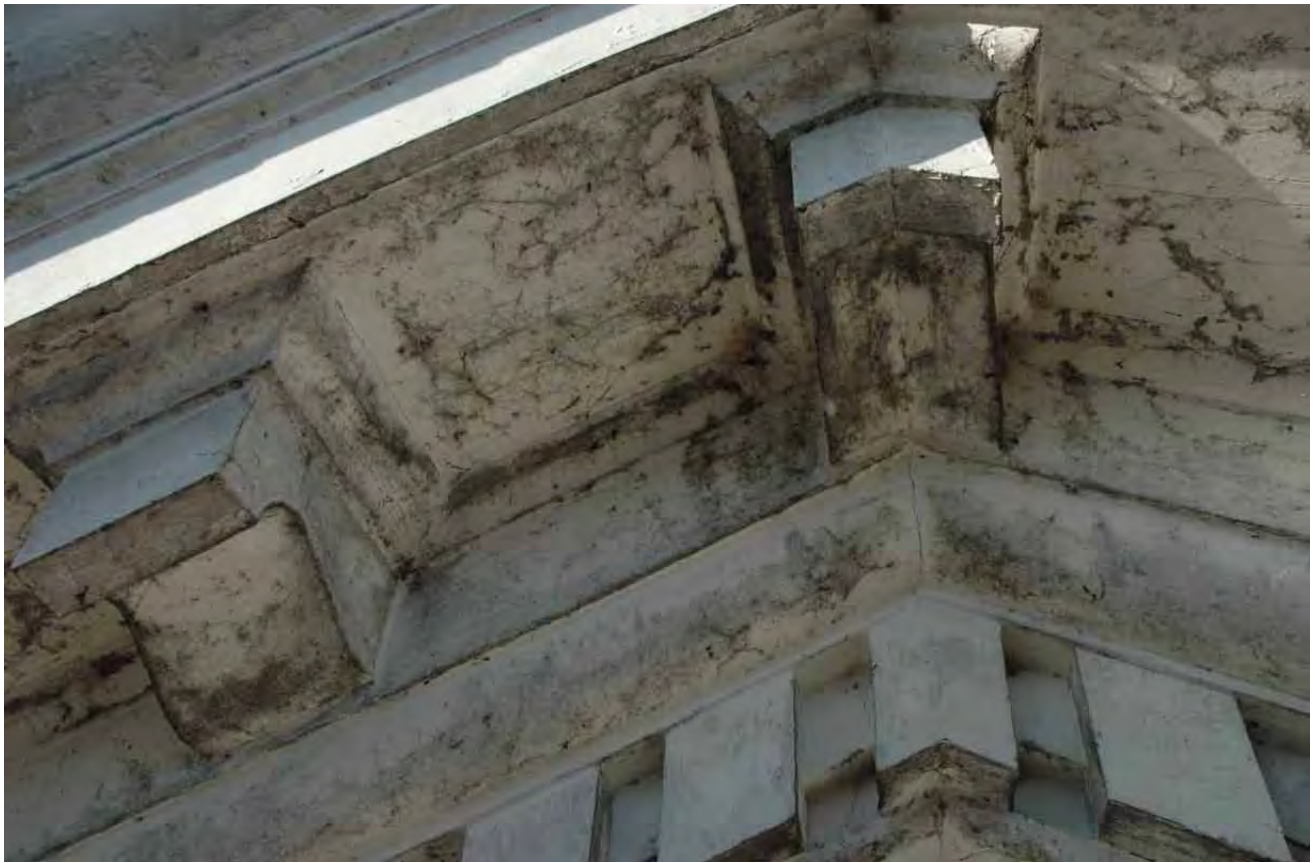
4. Deteriorated slope cornice with mold. This mold was prevalent throughout all cornices.
