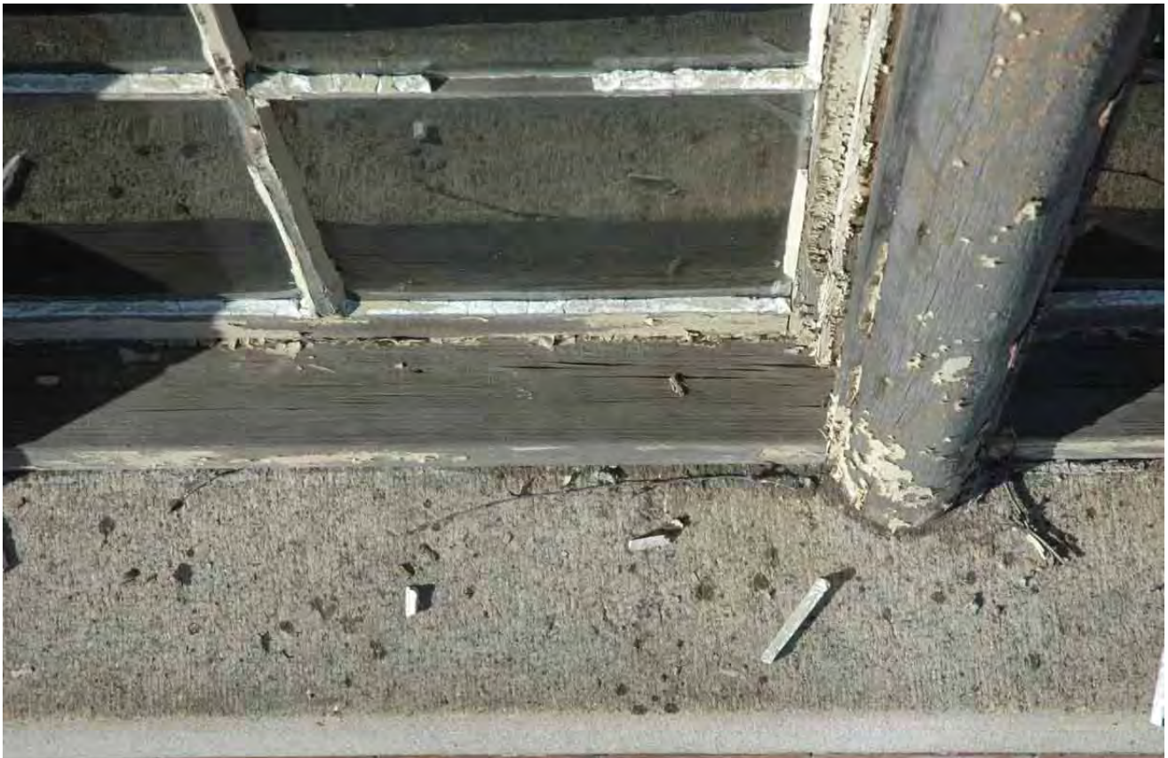
14. Severely Weathered Window Sill and Half-Round Mullion.
