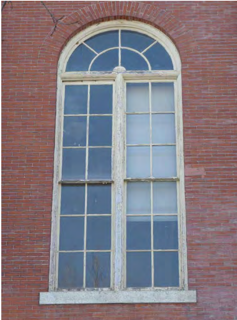
27. Pre-restoration round top window assembly showing severely weathered mullions, window sashes, sub-transom, frame and overlight.
