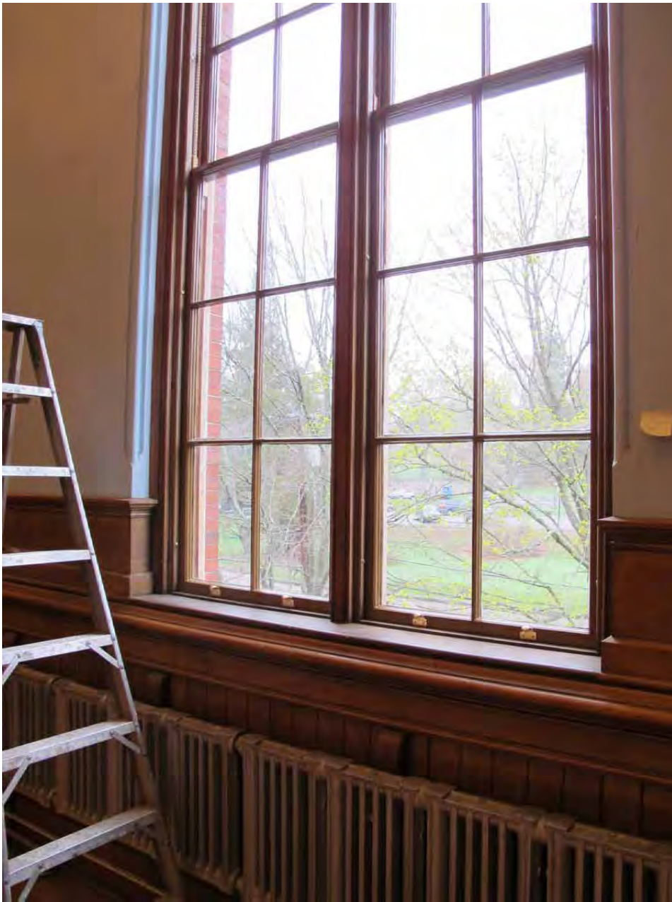
29. The interior of the mock-up was reviewed for paint colors, sash locks and sash lifts, sash chains and pulleys, weatherstripping, glazing appearance, and ease of operation.
