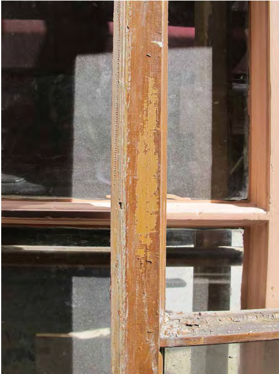
19. A number of different window sashes were inspected to confirm their original paint color.
