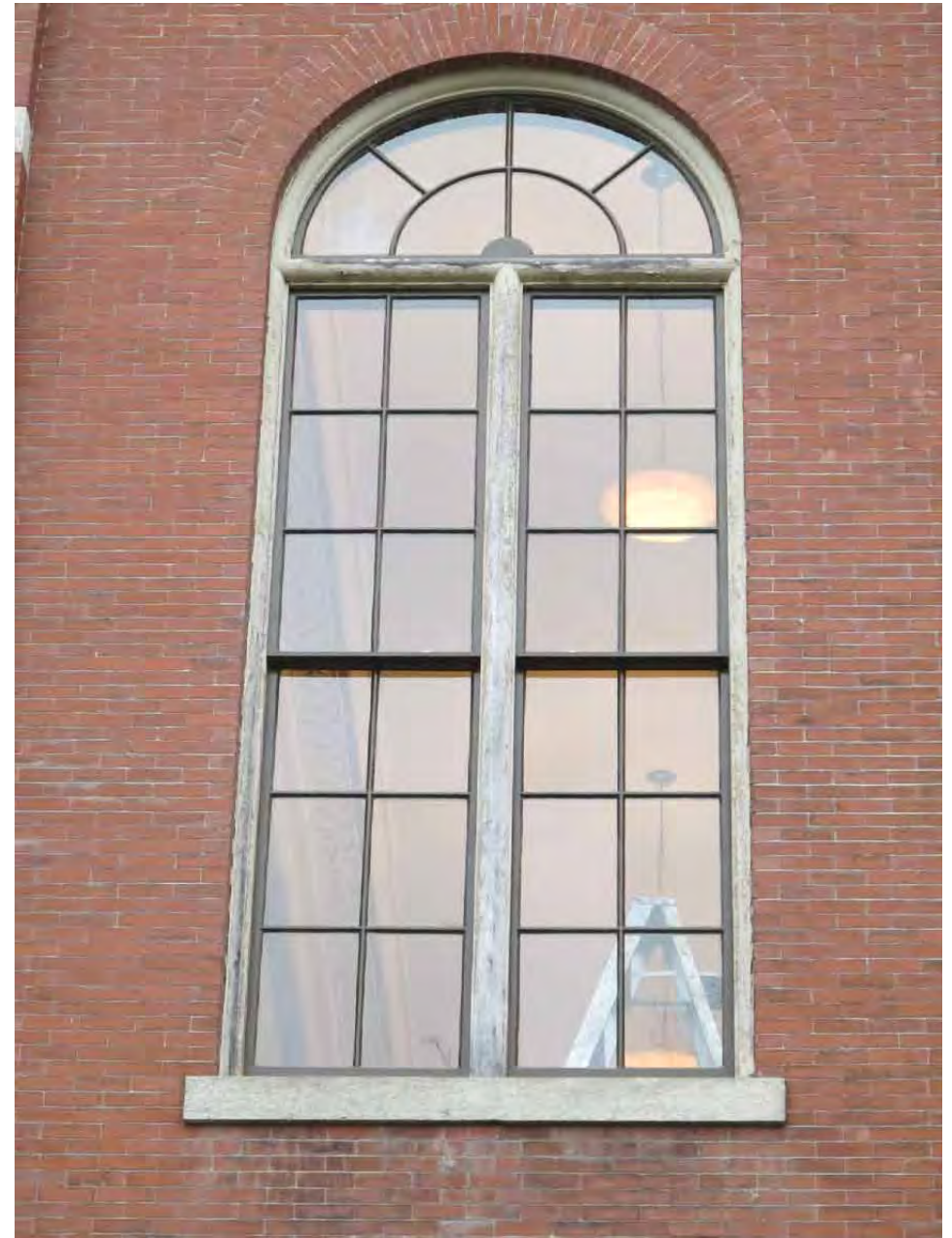
28. A window sash mock-up was installed for review by MK&A, the Town, and MHC, before authorizing a full-scale production effort at the woodwork shop and installation of completed units.
