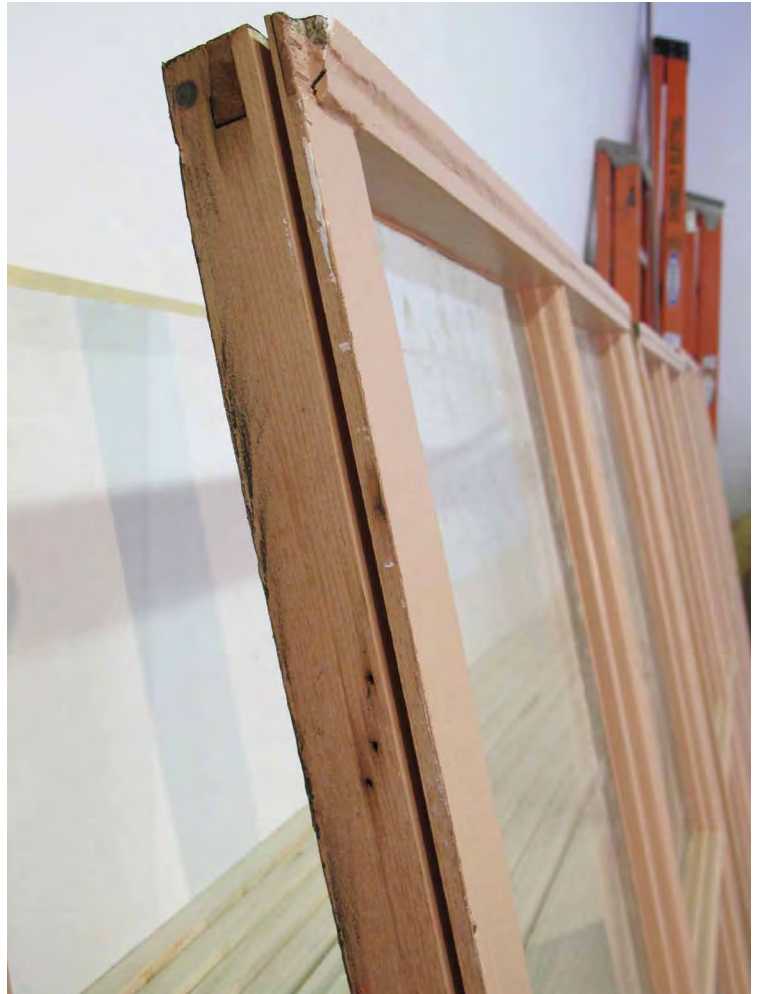
18. As part of the restoration work, kerfs were cut into the stiles of each sash to receive new metal weatherstripping.
