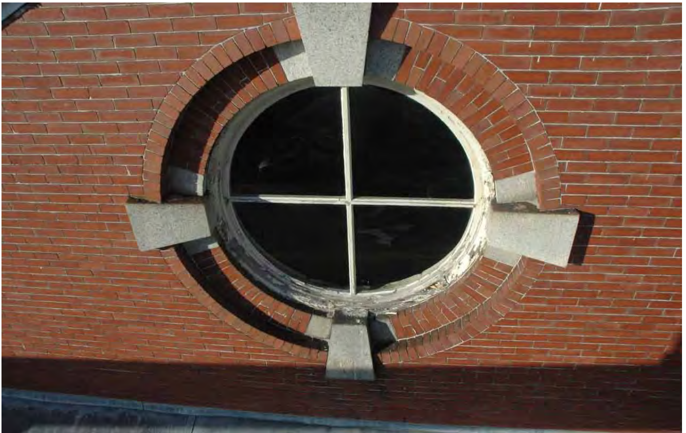
36. 20th Century Replacement Attic Sash Showing Severe Deterioration.
