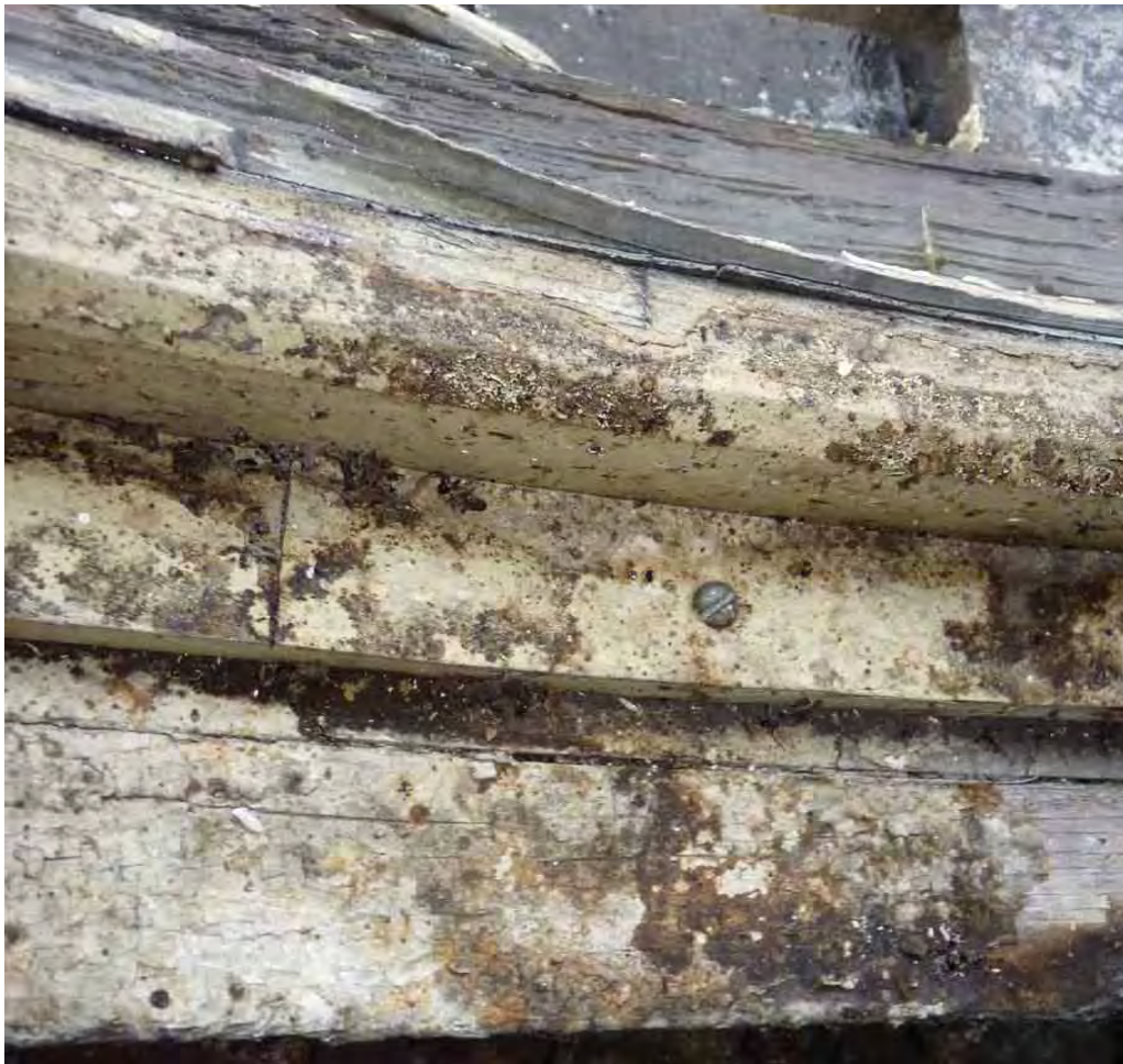
5. Deteriorated Interior of Circular Window Sill
