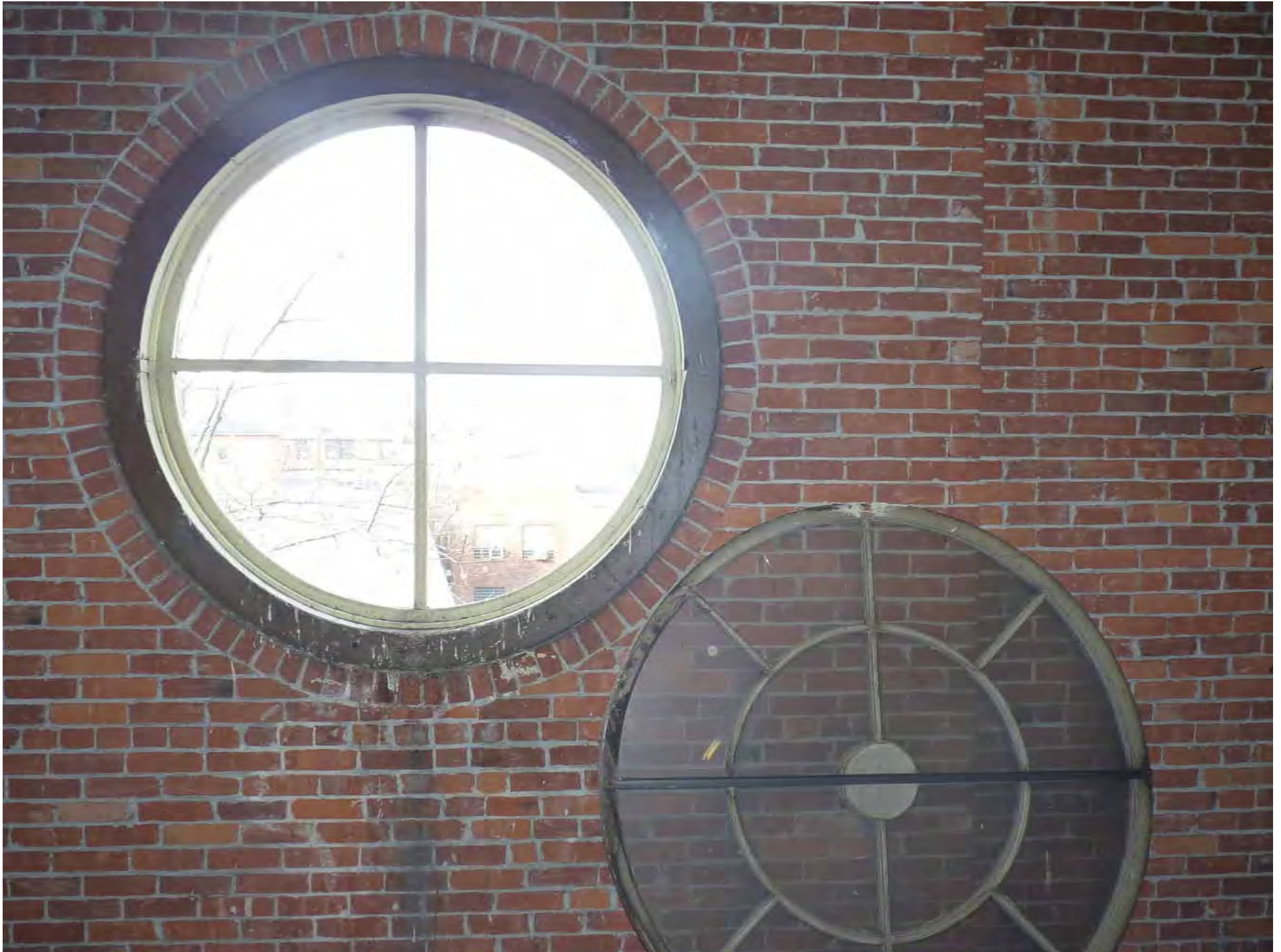
35. 20th Century Replacement Attic Sash with Original Severely Deteriorated Window Sash to Right, which was found in Attic.
