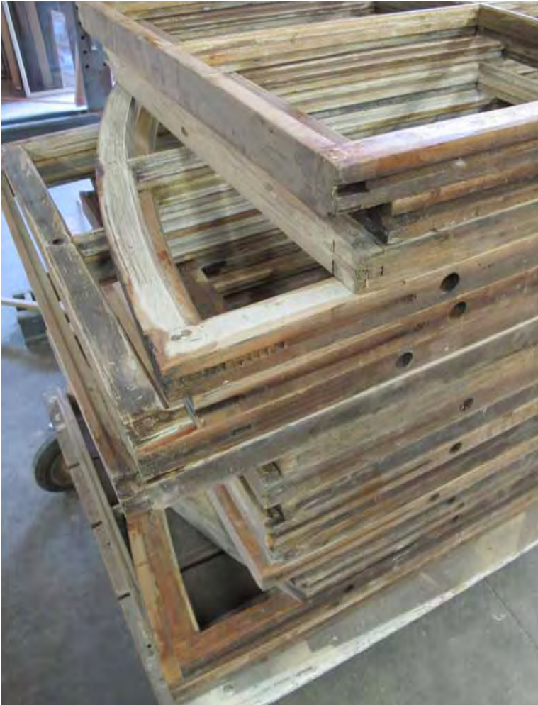
17. These window sashes have had loose connections mechanically repaired, and deteriorated wood areas repaired with epoxy wood consolidants and patching compounds.
