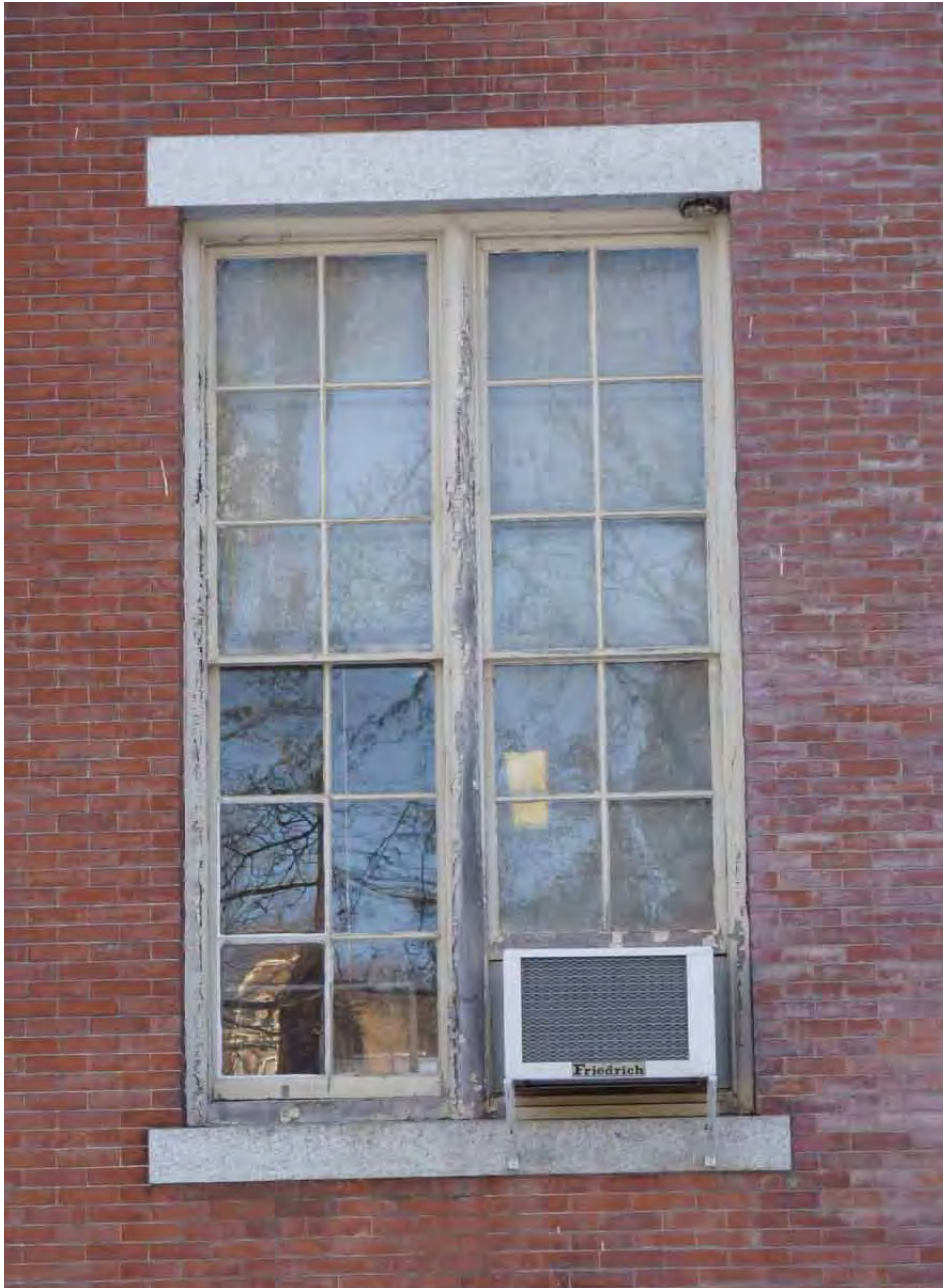
31. Pre-restoration window with window sashes, mullions, sills and frame all severely weathered.
