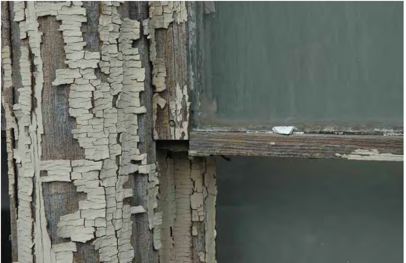
13. Closeup of Failed Meeting Rail
