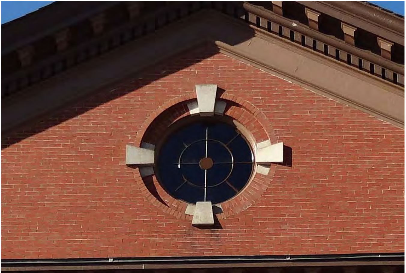
37. The original eastern round window had previously been replaced with a simplified new design. After restoration, this window was relocated to the more protected west end of the attic. The newly constructed round window was placed at the east end, which has more exposure to the elements.
