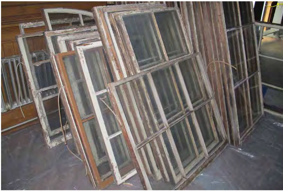
16. Once removed, window sashes were individually numbered to make sure they were reinstalled in the correct opening. Before being removed from the site, all glazing putty and glass was removed during an abatement process. Approximately two-thirds of all original glass was removed without breakage, and saved for reinstallation. W.W. Millworks performed the restoration of the windows in its shop.
