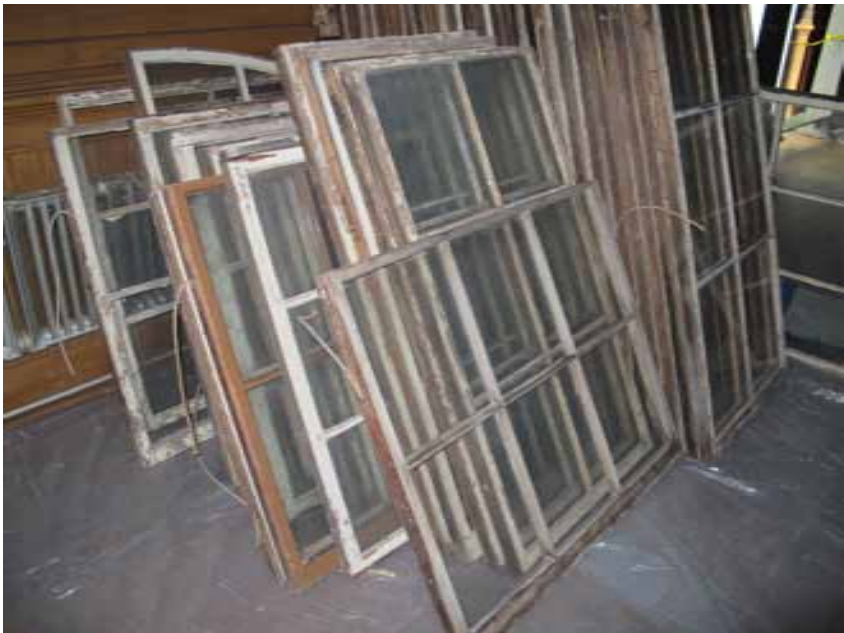
8. 2nd Floor Meeting Room: Once removed, window sash were individually numbered to make sure that they were reinstalled in the correct opening. Before being removed from the site, all glazing putty and glass were removed during an abatement process. Approximately two-thirds of all original glass was removed without breakage, and saved for reinstallation.
