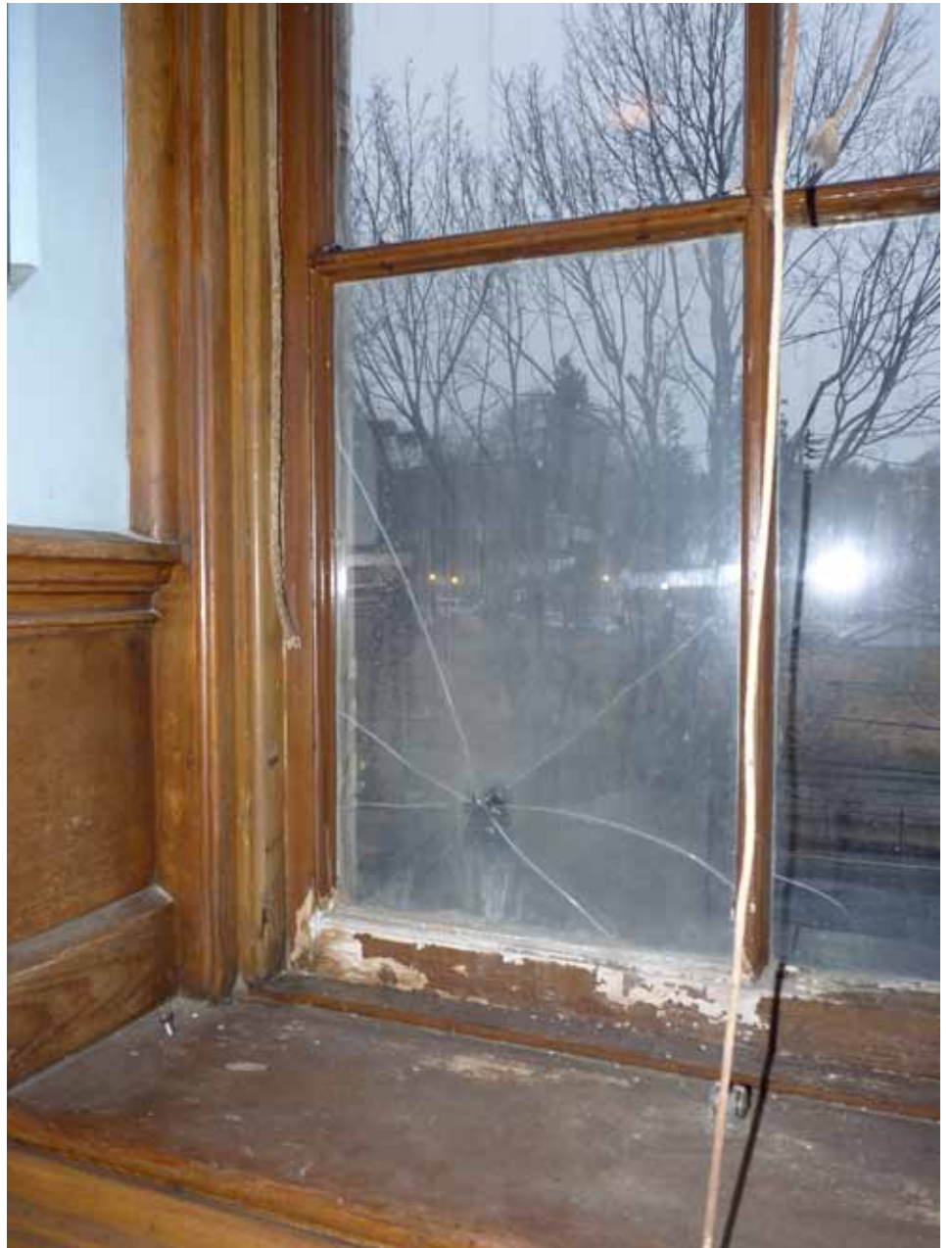
4. Typical 1st Floor Window (interior): window finish is water-damaged due to missing glazing putty, sash cords are broken, and there is glass breakage
