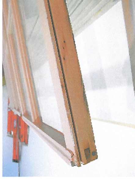
Kerfs are being cut into jamba's of sash to receive new metal weather-stripping
