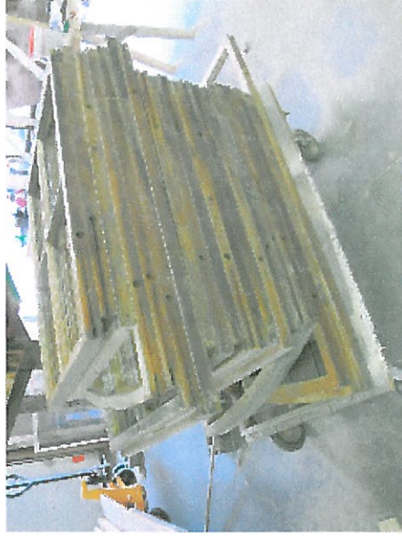
Appearance of sash after being stripped of paint & sanded
