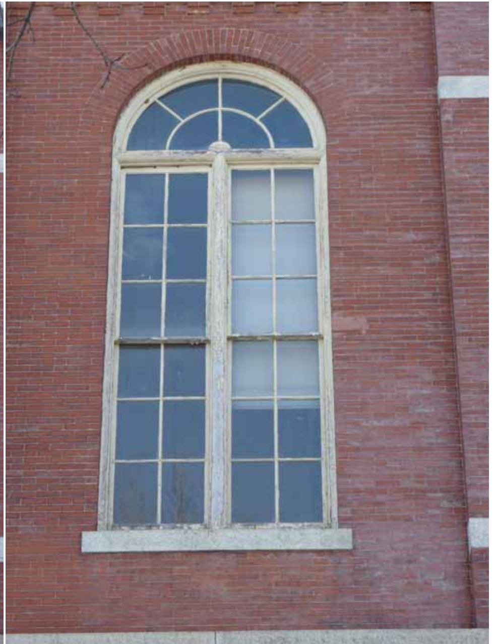
2. 2nd Floor Window N006, North Elevation: window sashes, mullions, sills, transom, frame, and overlight are all severely weathered
