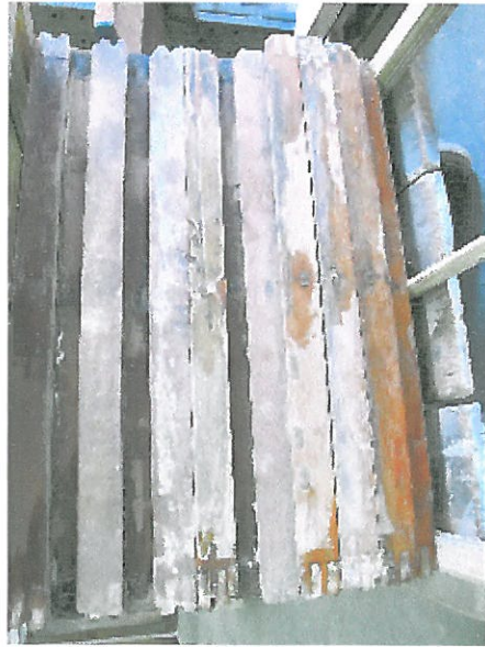
Epoxy repairs made to corner joints & mortise-and-tenon joints of window muntins
