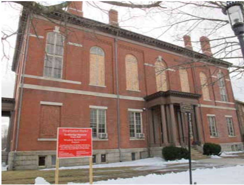
7. North Exterior Elevation: During the window removal process, wafer board sheets were installed in all window openings.
