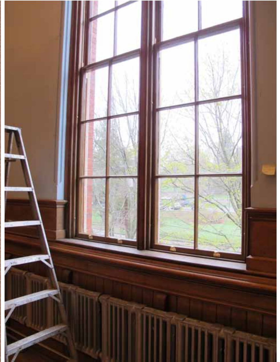
15. 2nd Floor Window N002, North Elevation, Interior View: The interior of the mock-up was reviewed for paint colors, sash locks and sash lifts, sash chains and pulleys, weatherstripping, glazing appearance, and ease of operation.
