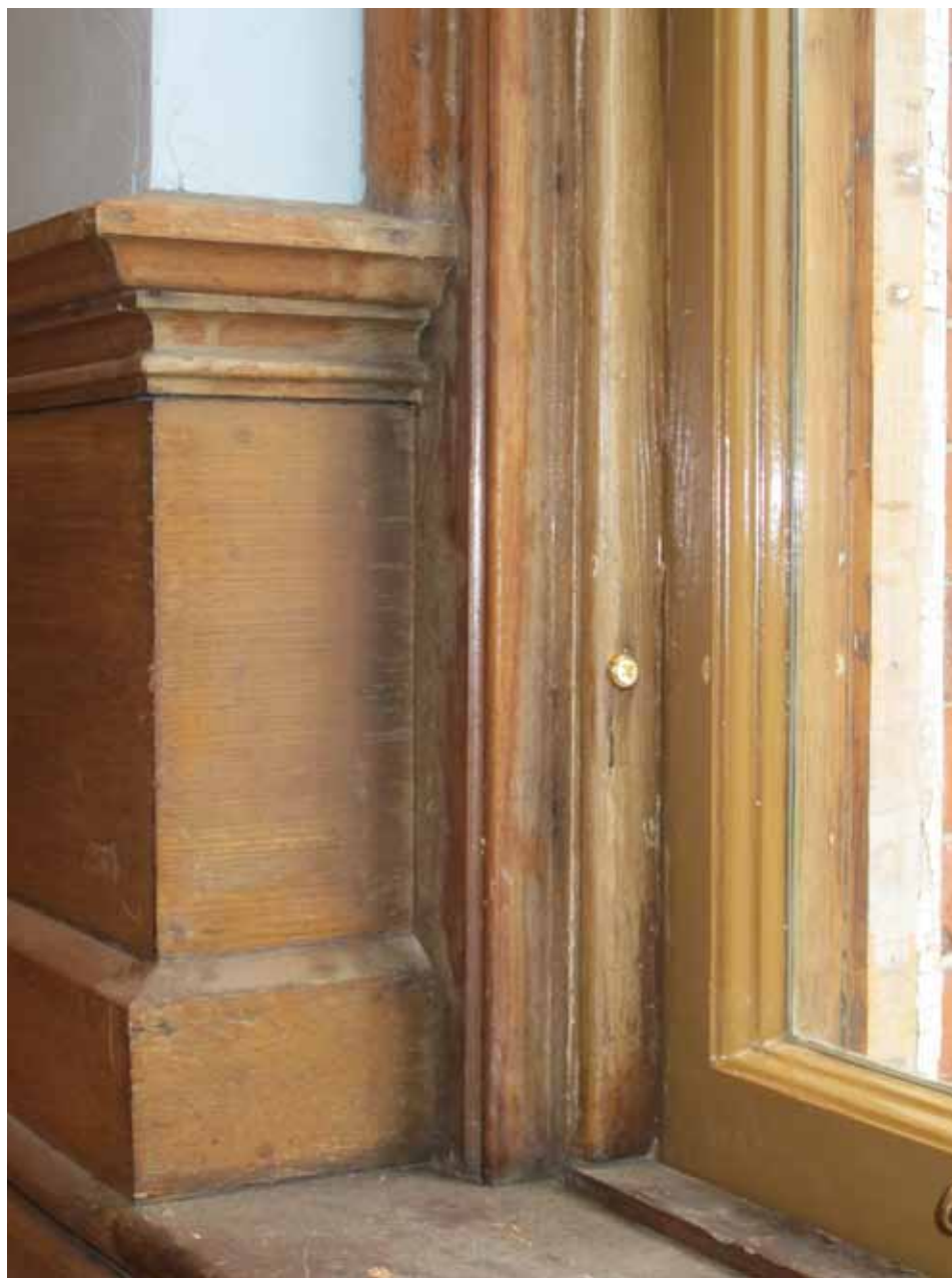
17. 2nd Floor Window N002, North Elevation, Interior View: The newly restored and painted window sashes complemented the finishes of the naturally finished wood of the adjoining window frame. The mock-up was approved by MK&A, as well as by representatives from the Town and the local Historical Commission.
