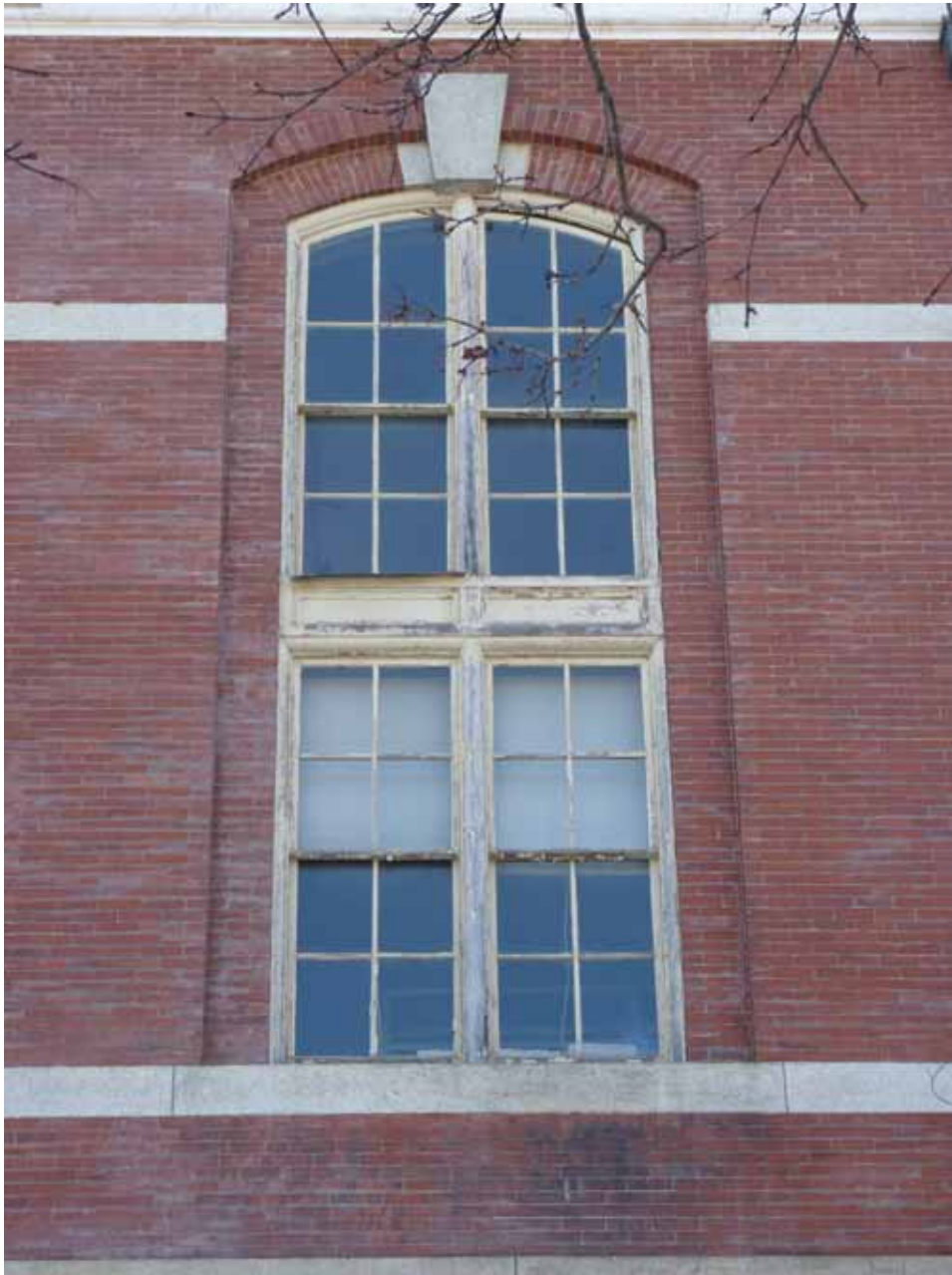
1. 2nd Floor Window N001, North Elevation: window sashes, mullions, sills, transom and frame are all severely weathered
