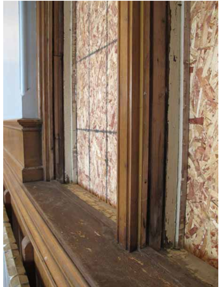
9. 2nd Floor Meeting Room: Wafer board was secured to the window frame from the outside of the building. Interior window stops were also numbered for reinstallation into the correct opening.
