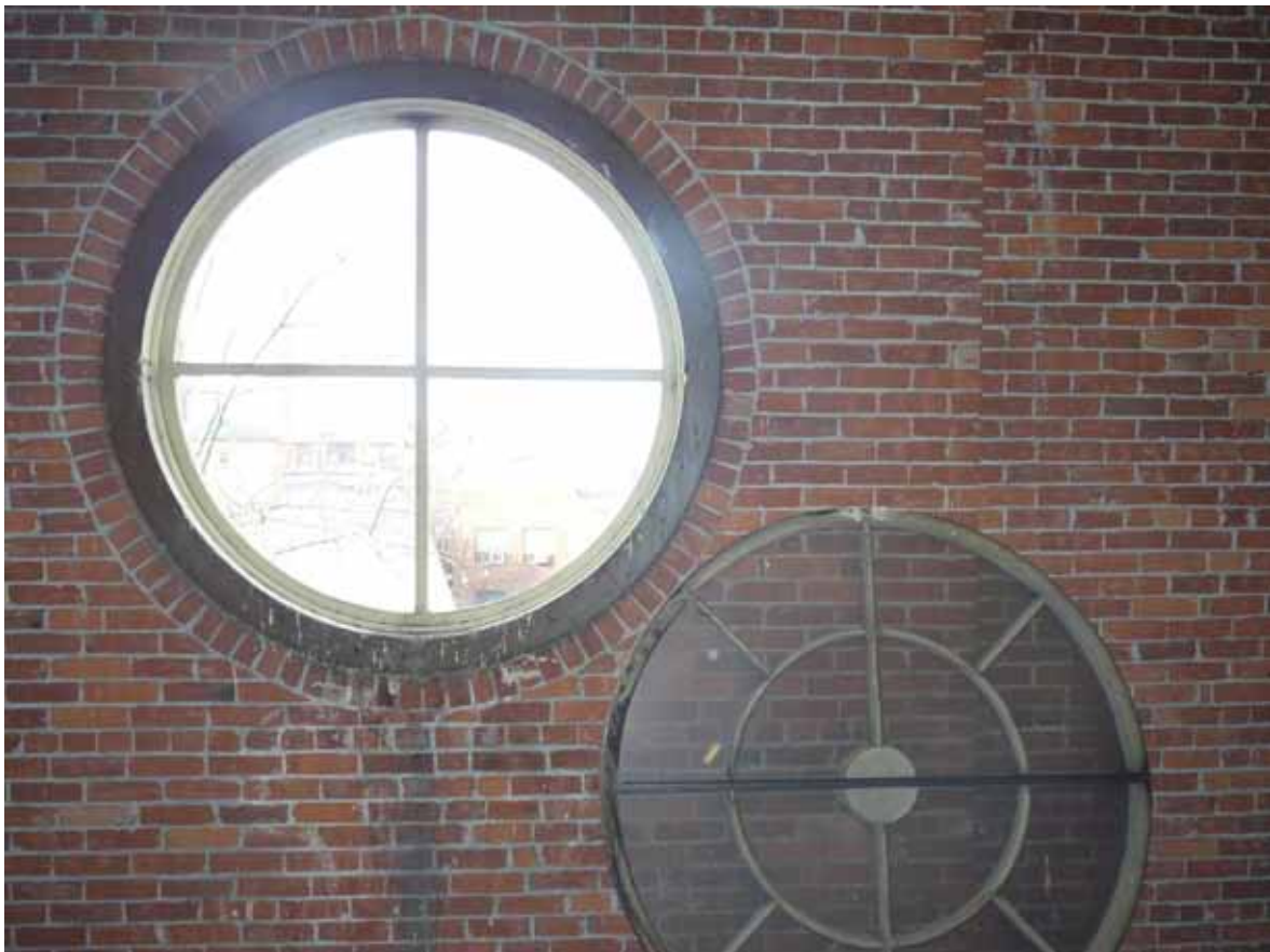
6. Attic Window W001, West Elevation: original severely deteriorated round sash is resting on the floor, below a simplified replacement unit.
