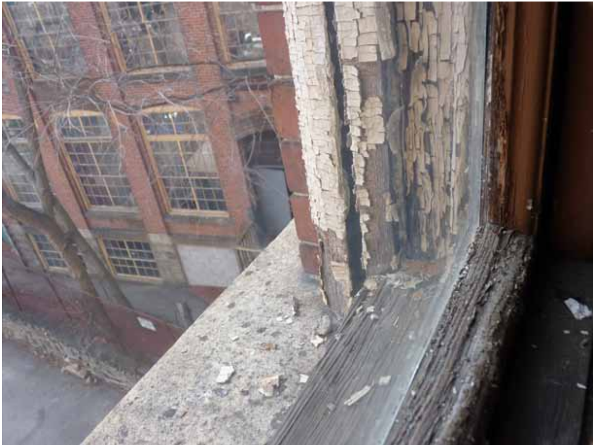
5. Typical 2nd Floor Window Sill: window sill, frame, and brick moulding are all severely weathered at south elevation; north elevation sills were in much better condition
