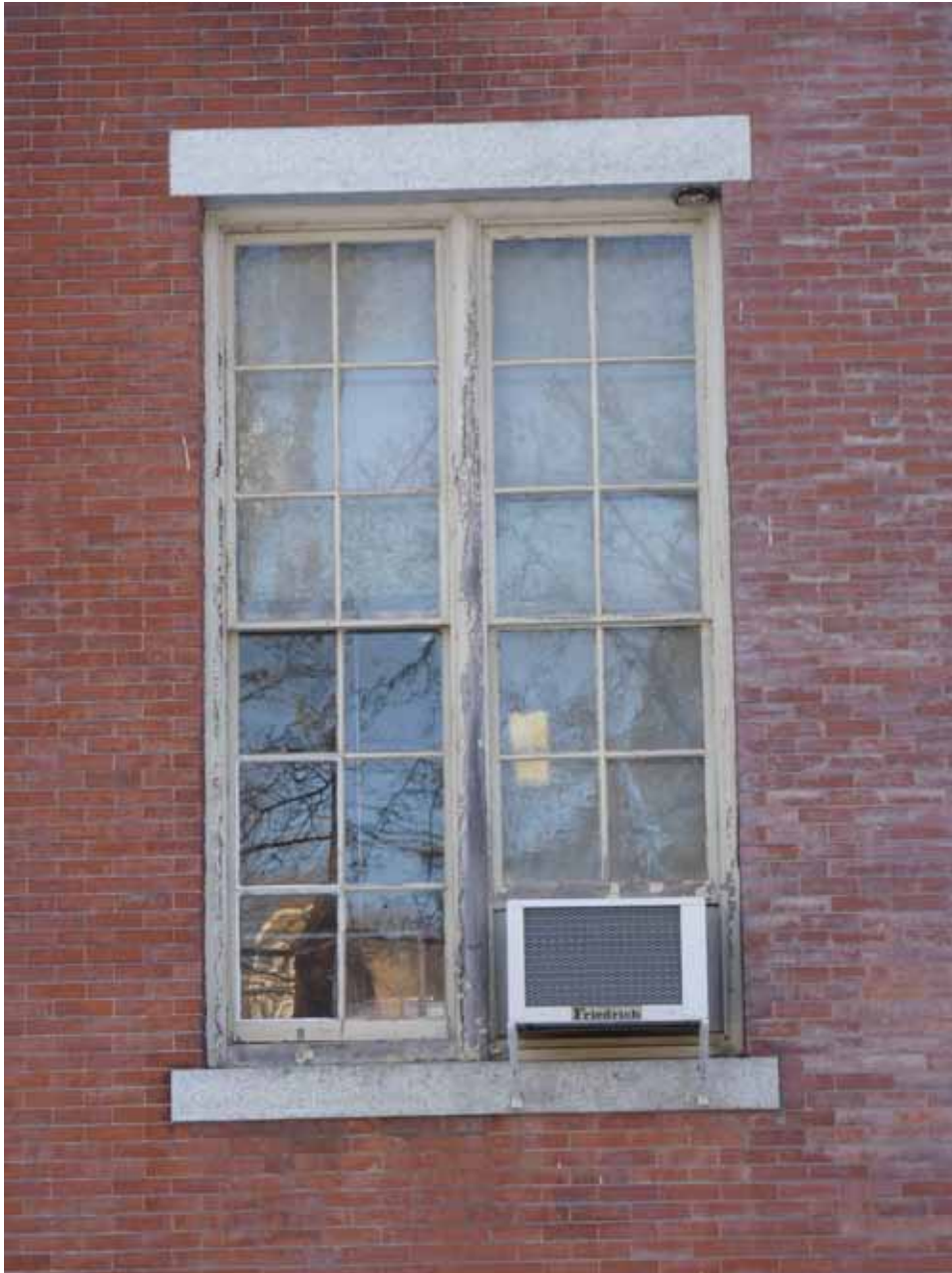
3. Typical 1st Floor Window (exterior): window sashes, mullions, sills, and frame are all severely weathered
