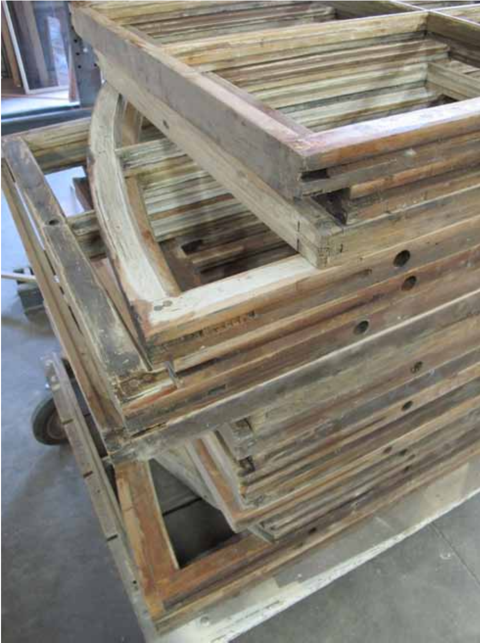
10. Wojciech Wasilewsky Woodwork Shop: These window sashes have had loose connections mechanically repaired, and deteriorated wood areas repaired with epoxy wood consolidants and patching compounds.
