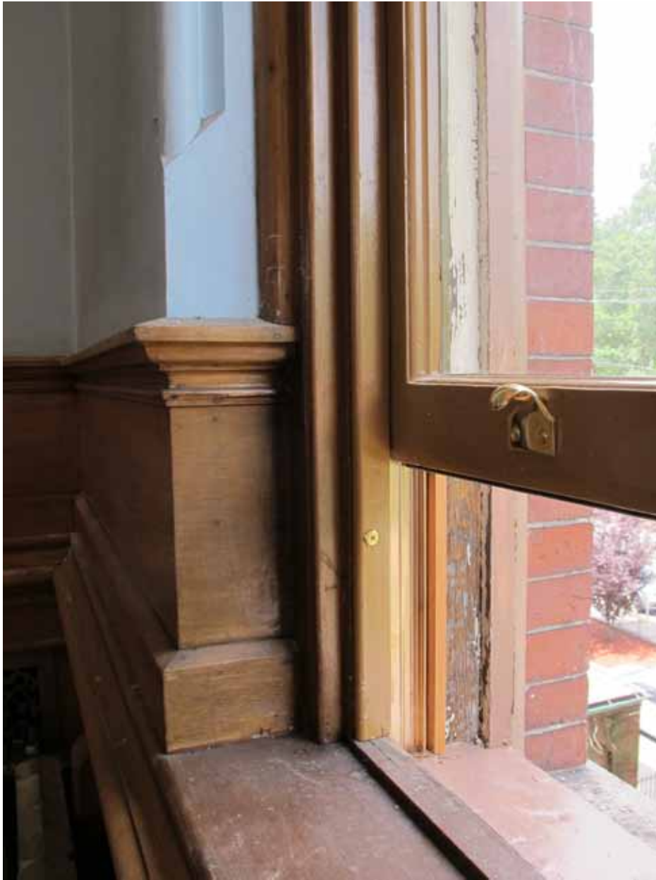
22. North Window Jamb and Sill at 2nd Floor : The wood surfaces of the interior window frame, sill and adjoining wainscot were not part of the work scope. The wood window stops were part of the work scope and were painted to match the restored sash. Visible in the photo are the new sash lifts, brass grommets on the window stops, and the new metal weather-stripping. The exterior wood window trim will be painted as part of the work scope.
