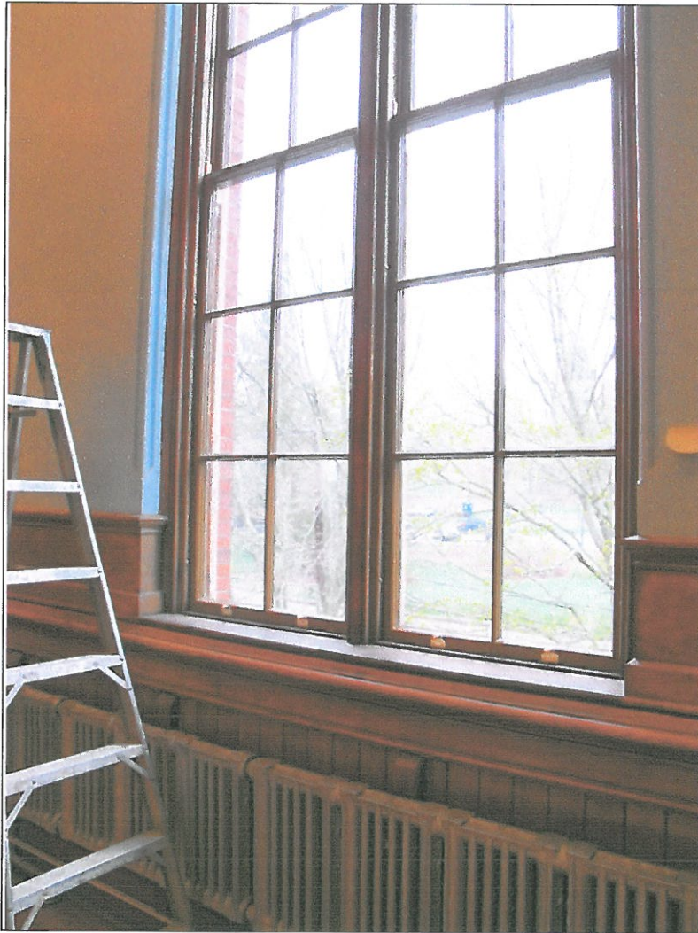
Bottom of window sash showing new sash lifts and reinstalled original window glass
