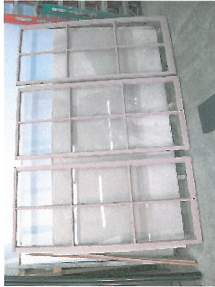
Stripped, sanded, primed & painted sash, ready for finish coat of tinted varnish
