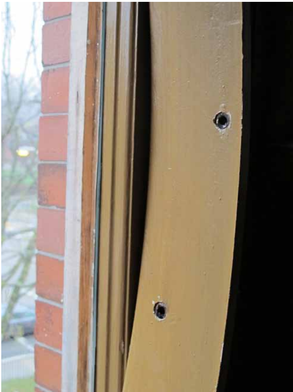
16. 2nd Floor Window N002, North Elevation, Interior View: A curved section of window stop taken from the head of one window was placed against the stile of the mock-up window. It was a very close match to the original finish on the curved stop, which had never been over-painted.
