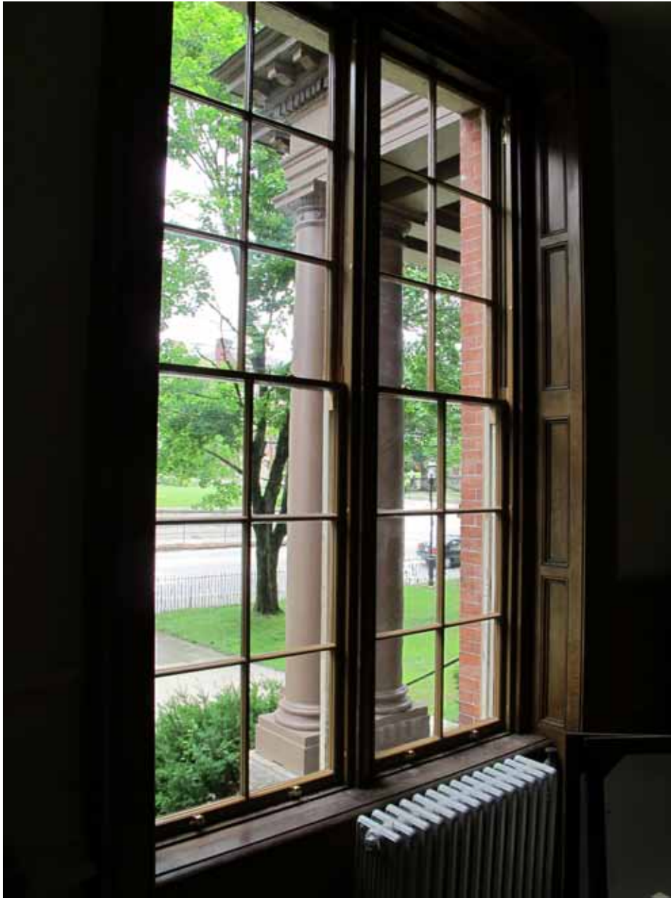
20. North Interior Elevation, 1st Floor Offices: The operation of the restored window sashes is relatively easy, considering that the sash weights only exist at the masonry opening side of each window, and not within the central vertical mullion. The narrow proportions of the windows probably make this possible.
