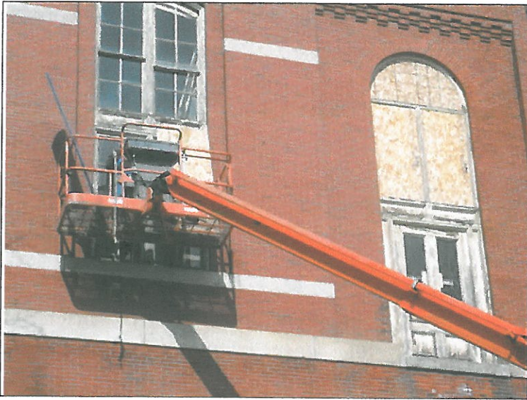
A Campbell Construction worker at Memorial Town Hall measures a window before boarding it up and removing it for restoration. Photo Credit: Deborah Gauthier
