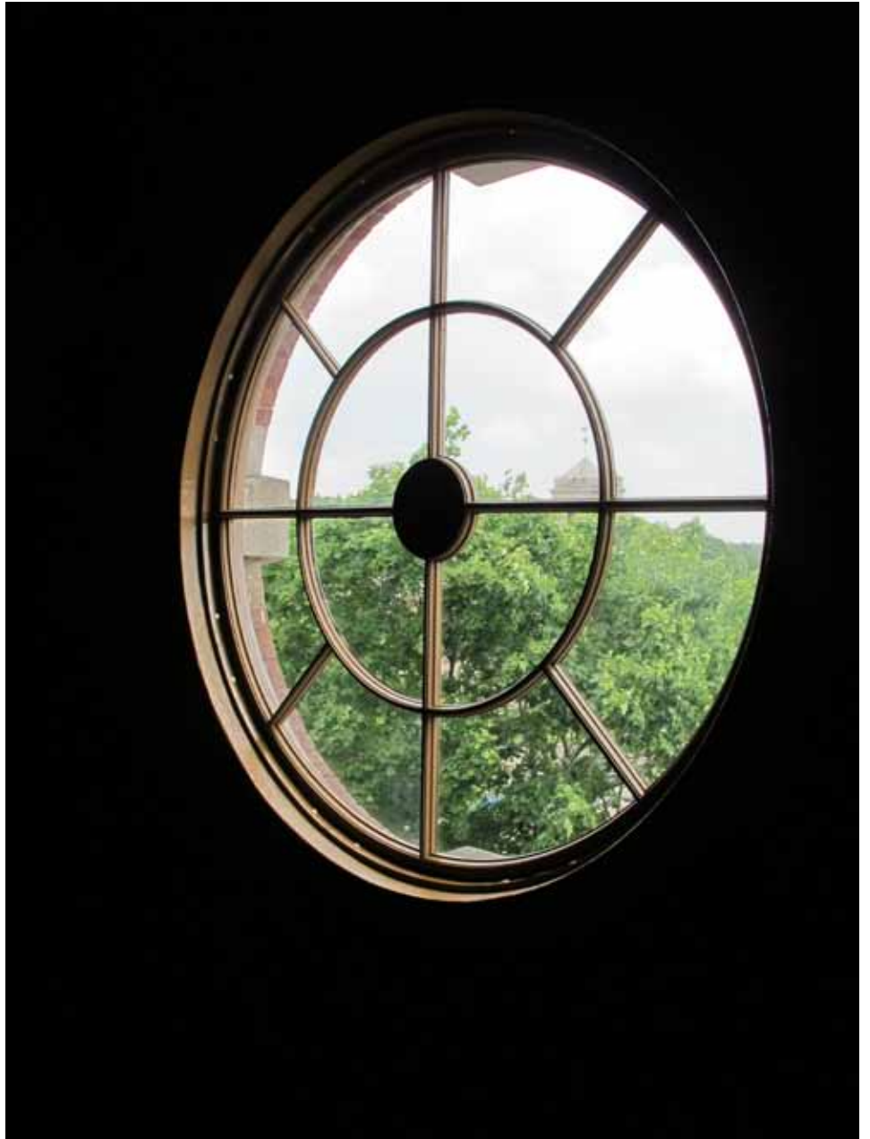
21. Interior Elevation of Round East Attic Window: The original eastern round window had previously been replaced with a simplified new design. After restoration, this window was relocated to the more protected west end of the attic. The newly constructed round window was placed at the east end, which has more exposure to the elements.
