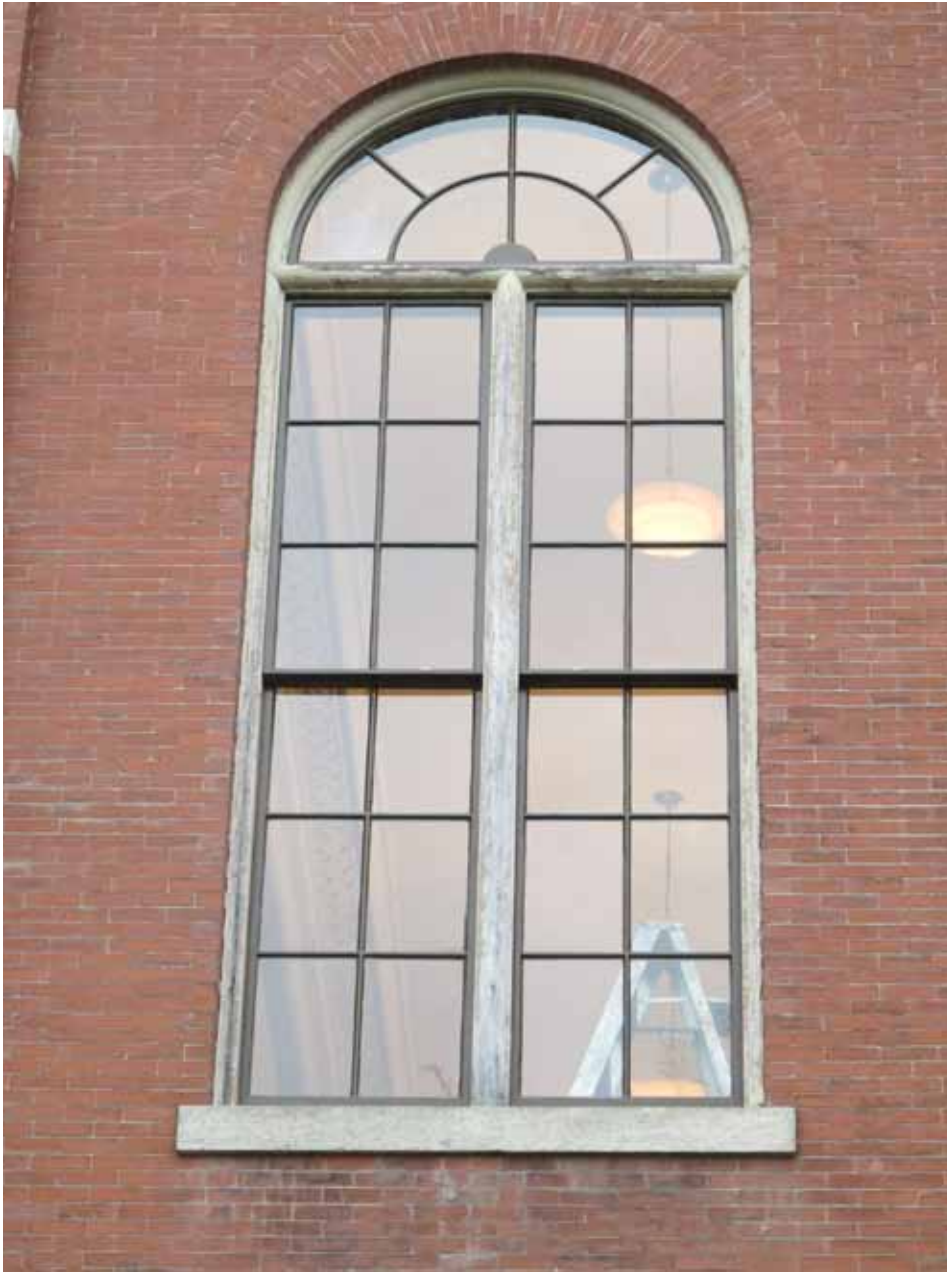
14. 2nd Floor Window N002, North Elevation, Exterior View: A window mock-up was installed for review by MK&A, the Town, and MHC, before authorizing a full-scale production effort at the woodwork shop, and installation of completed units.
