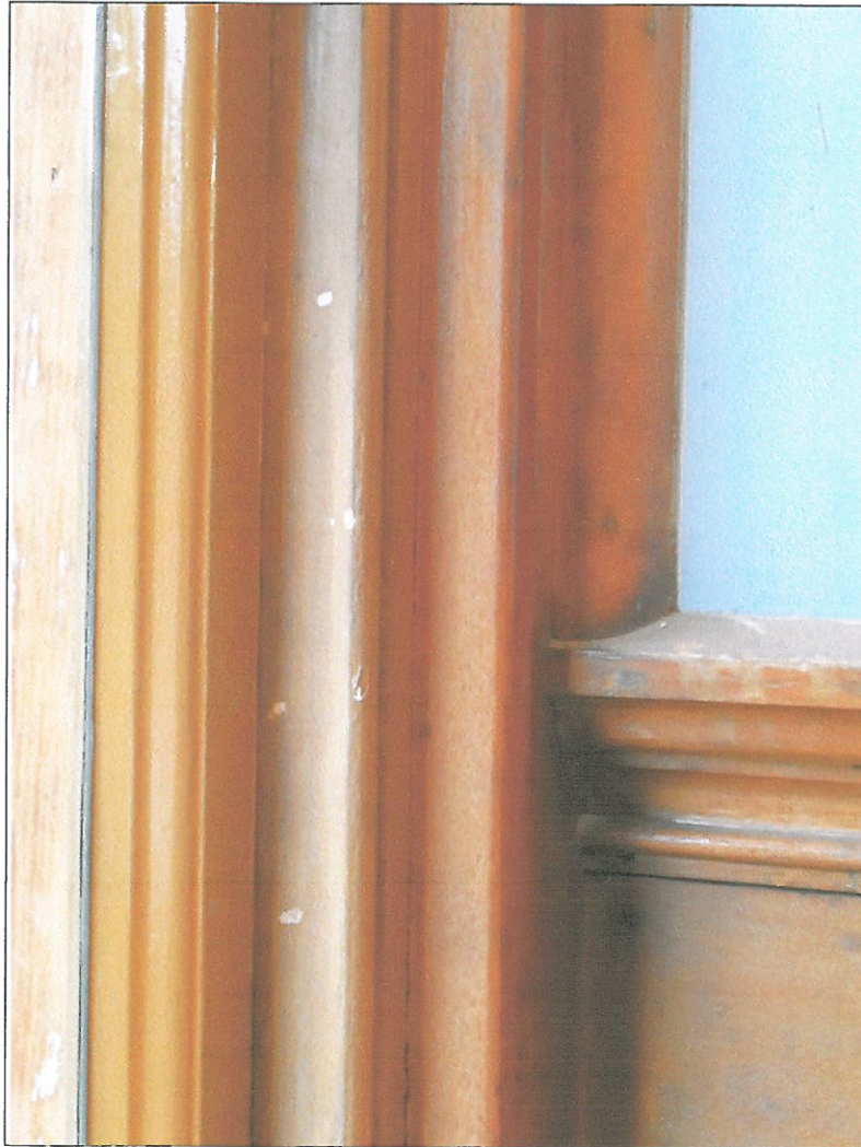
Painted window sash adjacent to reinstalled jamb stop (yet to be painted to match sash), with adjoining wood trim (existing clear varnish finish)
