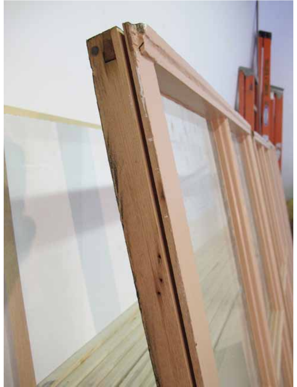
11. Wojciech Wasilewsky Woodwork Shop: As part of the restoration work, kerfs were cut into the stiles of each sash to receive new metal weatherstripping.
