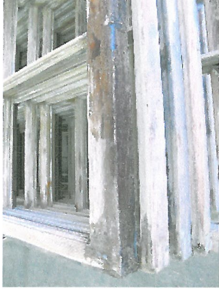
Dark areas of wood on top sash indicate epoxy repairs have been made to that area
