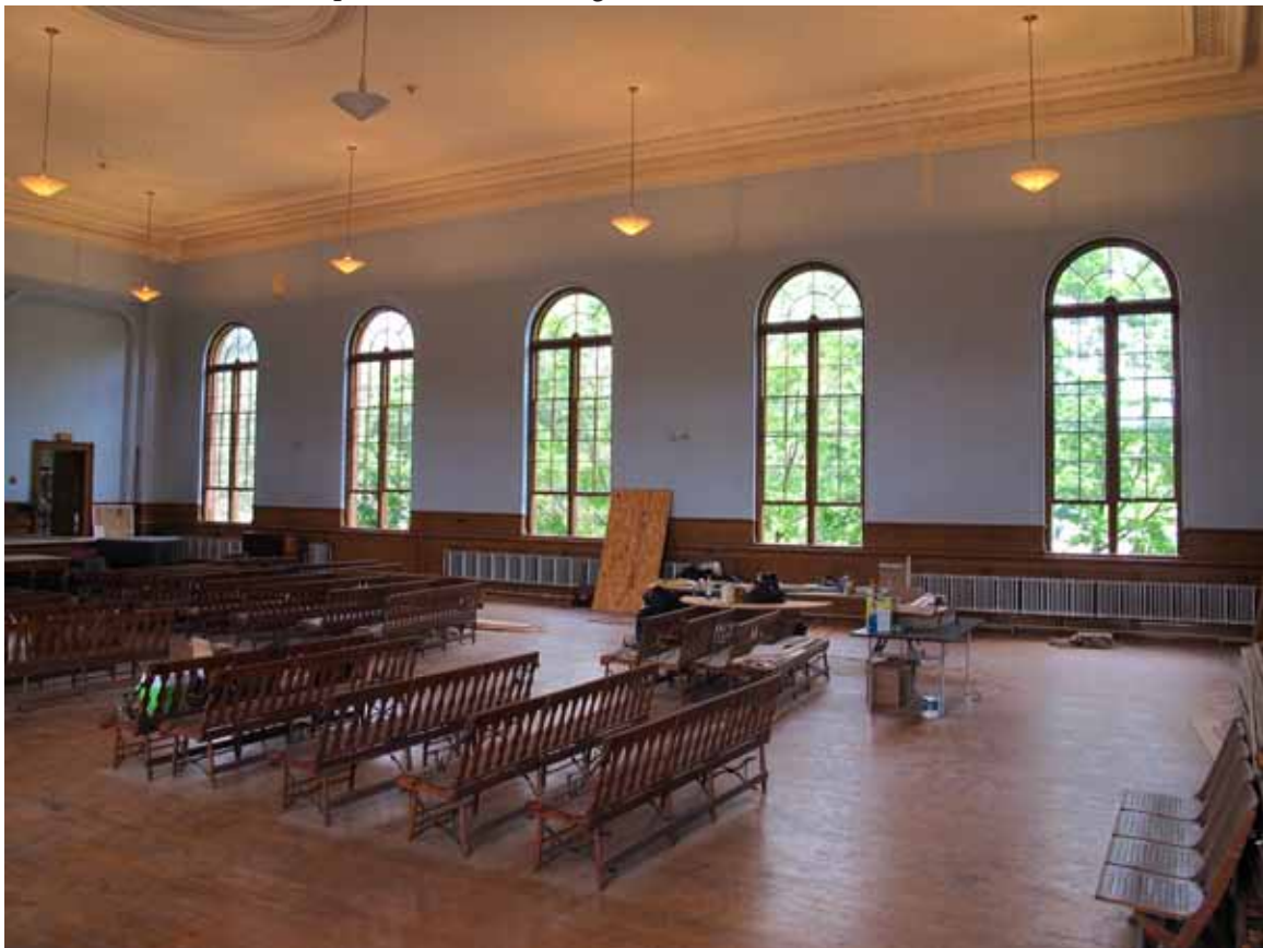
19. North Interior Elevation, 2nd Floor Meeting Room: From the interior, the cleaned glass offers a much greater transparency of light. The lower sashes are all operable, while the upper sashes are fixed in-place, to reduce air infiltration and energy loss.
