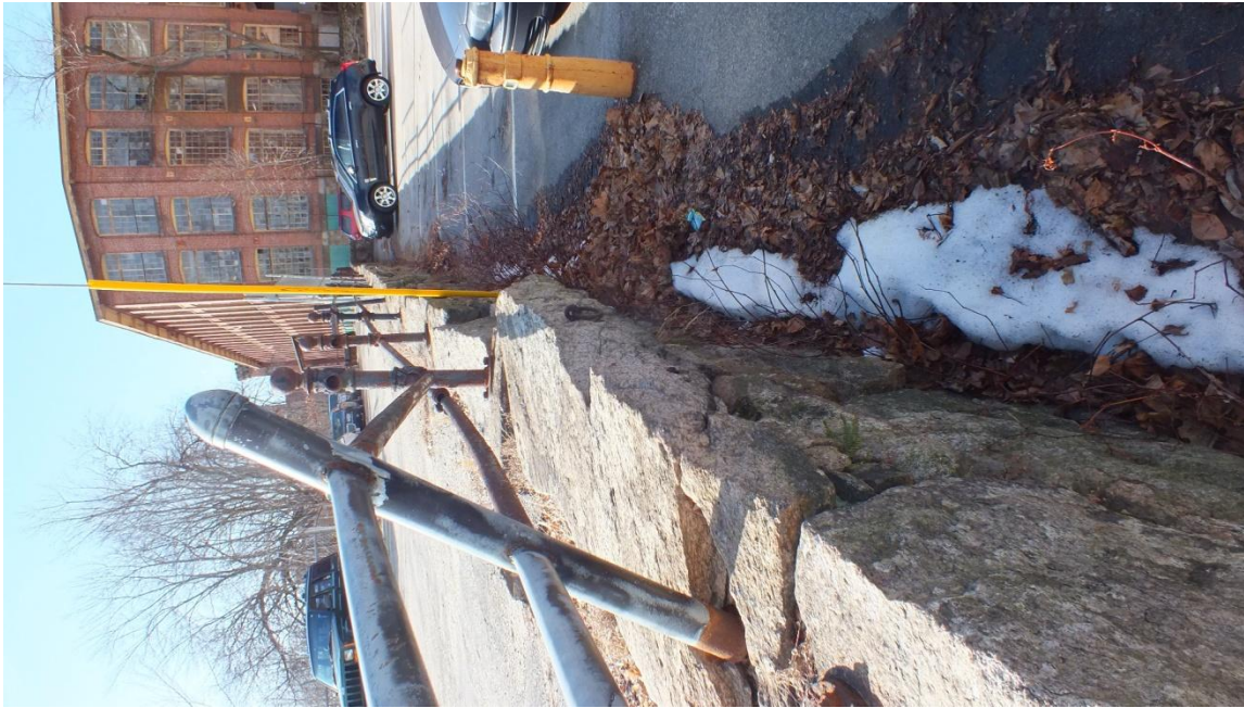
9. Retaining wall along south property line viewed from east. Coping dislocated by impact on railing.
