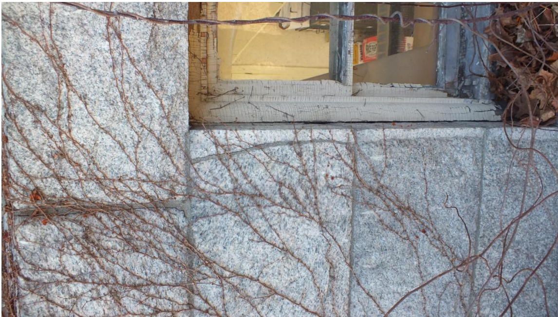
6. Cracked stone jamb at east elevation on left side of first window from south.
