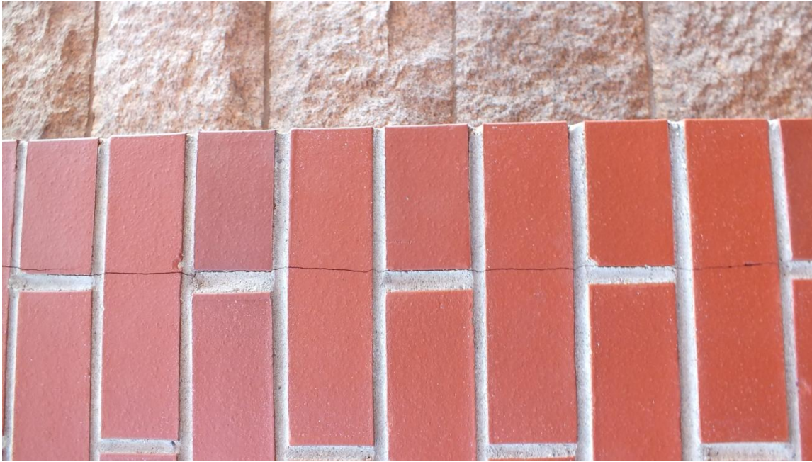
5. West chimney west face crack at ground level.
