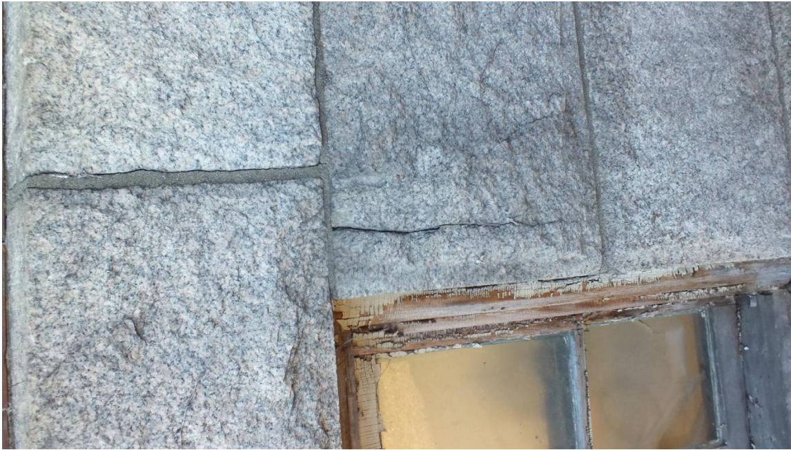
7. Cracked stone jamb at east elevation on right side of first window from south.
