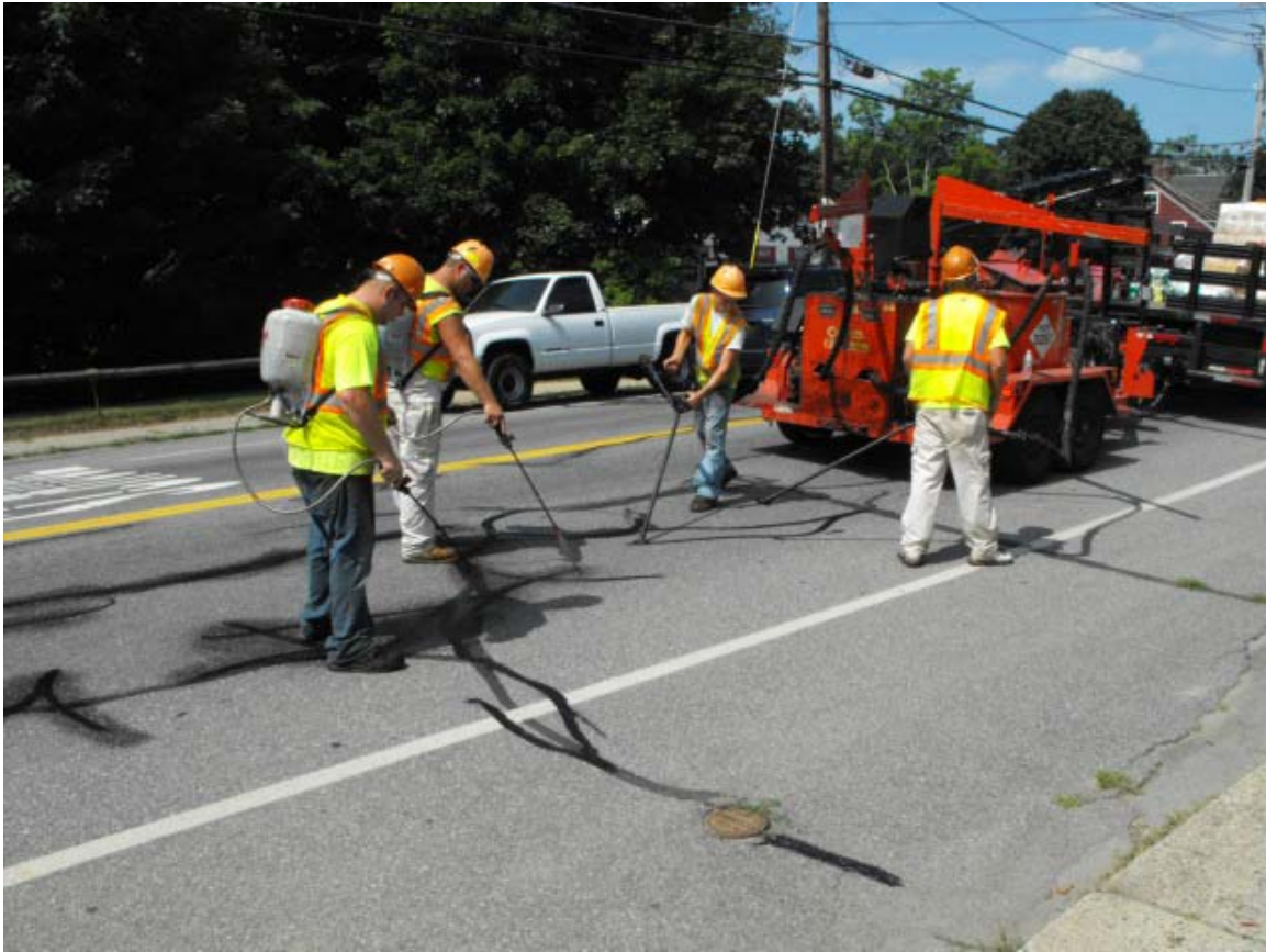
AnnSeal employees of Johnson City, NY fill seal on Linwood Avenue in Whitinsville.
