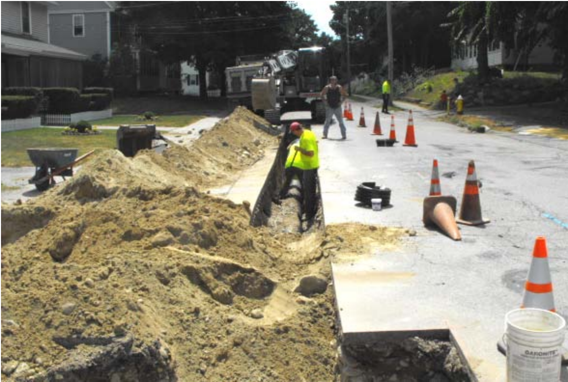
Employees of Sequoia Construction install new drainage piping on Crescent Street
